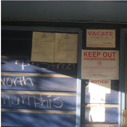
Figure 2.8 Condemned Home in N. Memphis, 2011. Photo by Neil Parrish
