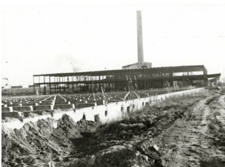
Figure 2.4 Firestone Plant Construction (Image Owner: Memphis Public Library)
