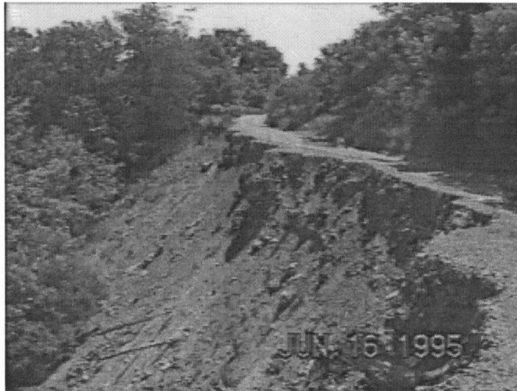
Figure 3-10 Slope Prior to Removal of Vertical Section
