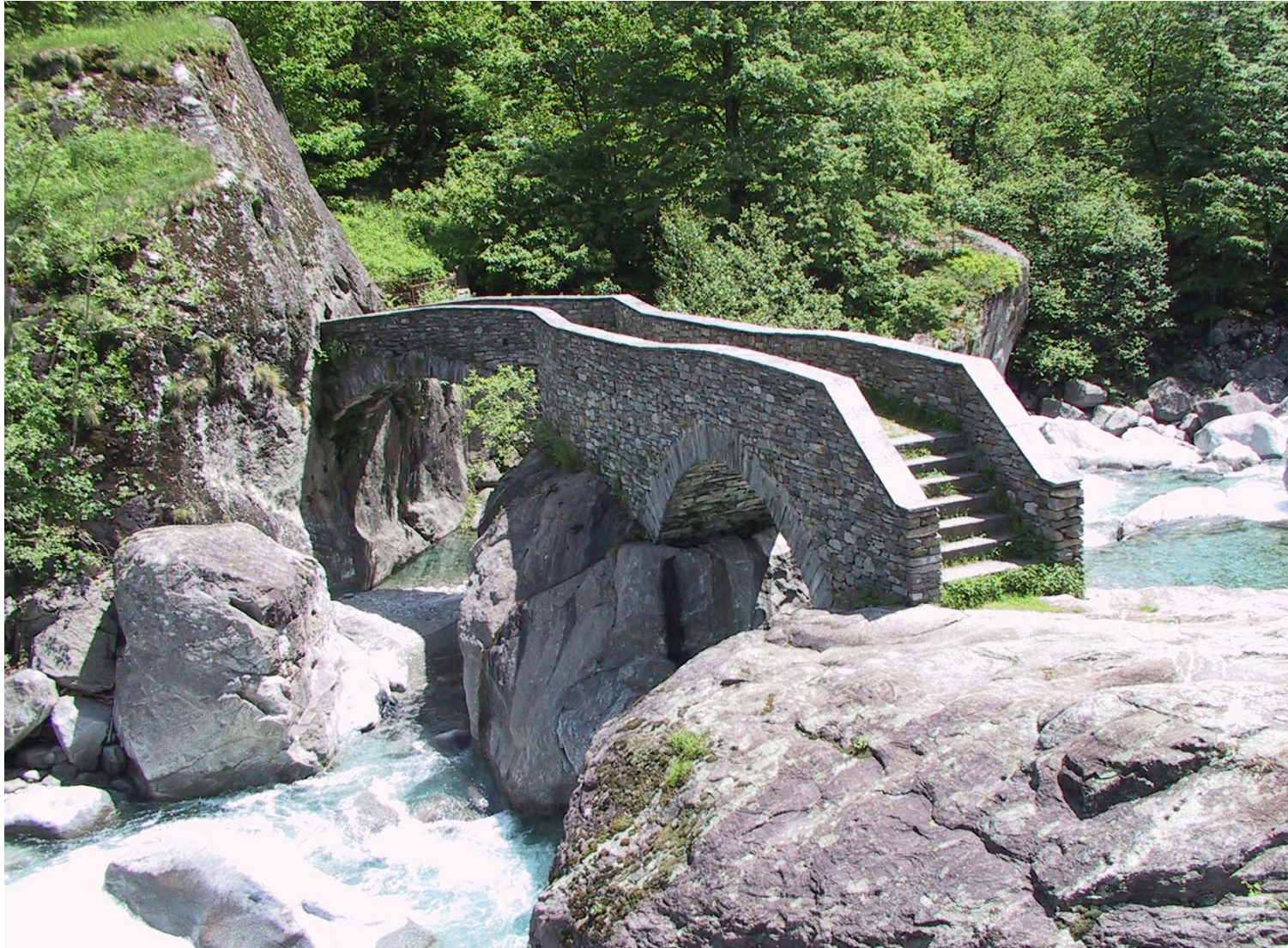
Fig. 1: Stone footbridge in Vallemaggia district, Ticino, Switzerland
