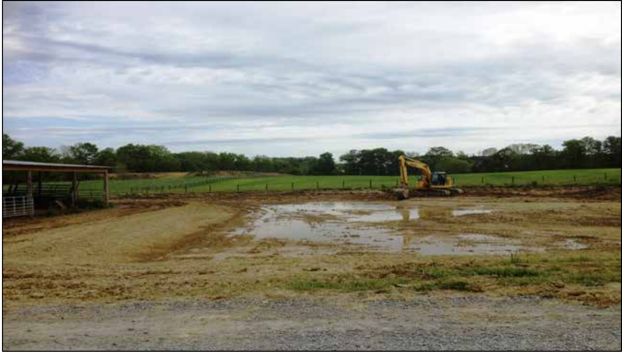
Figure 2.10 Constructed wetland underway (Ludwig, 2011).
