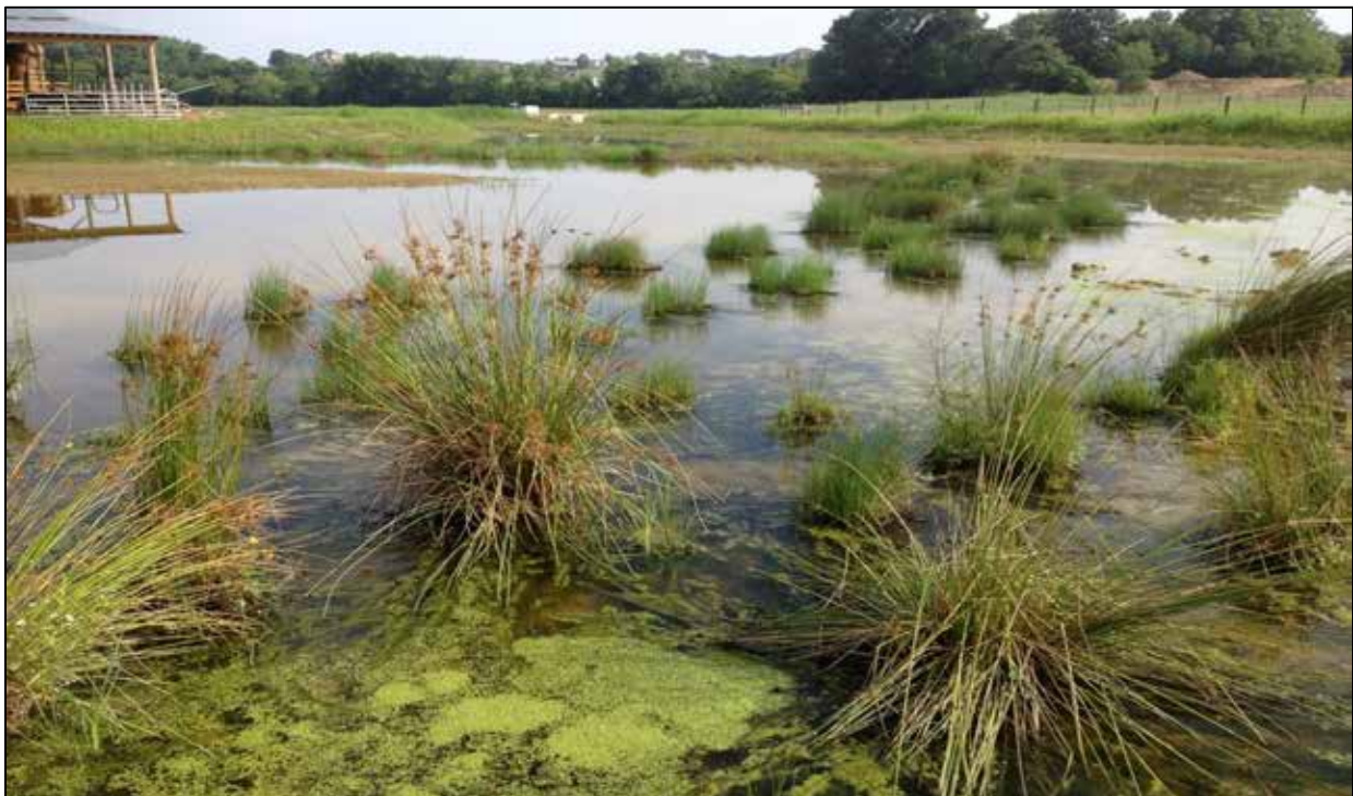
Figure 2.11 - Constructed wetland after with wetland plantings (Ludwig, 2011).
