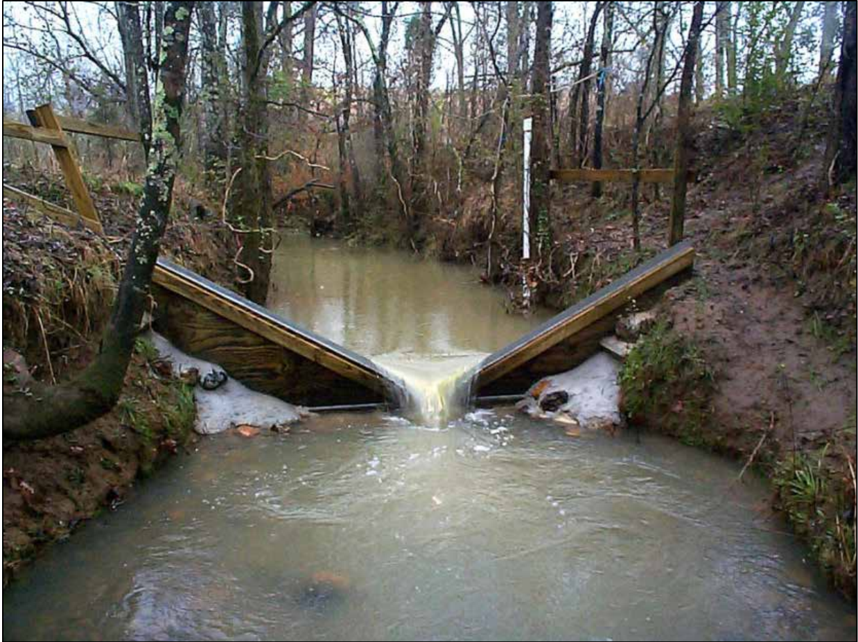
Figure 2.7 - Farm Stream (FS-2) -120 degree V-notch weir.
