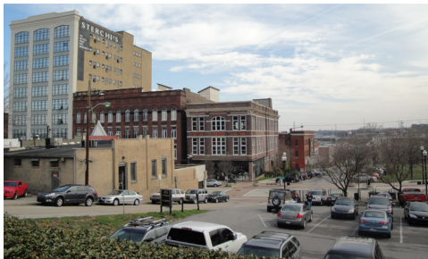
Figure 3.11: Existing Site Condition From The Crown Plaza Hotel
