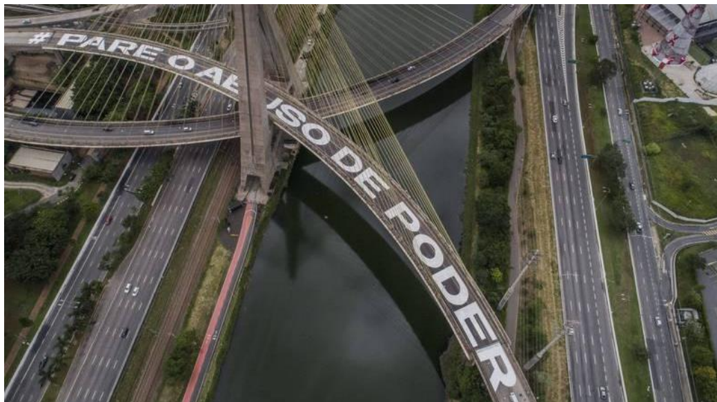
Figure 158. #Pare O Abuso De Poder (Stop Abuse of Power) Street Mural
