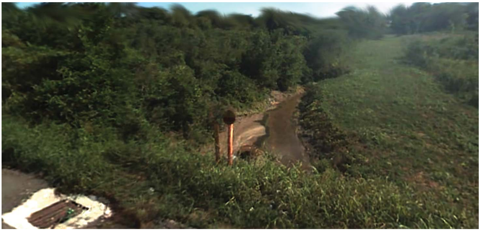
EXISTING STORM WATER DRAINAGE Source: google maps
