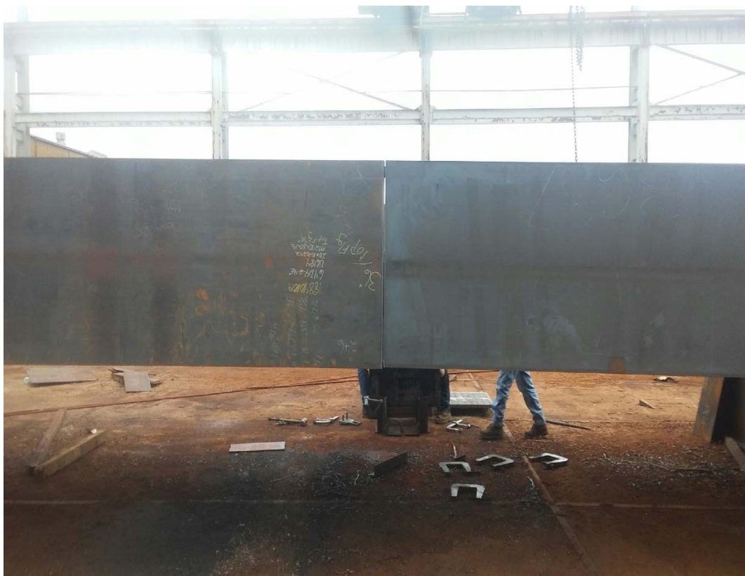
Figure 16: Beginning of girder laydown procedure
