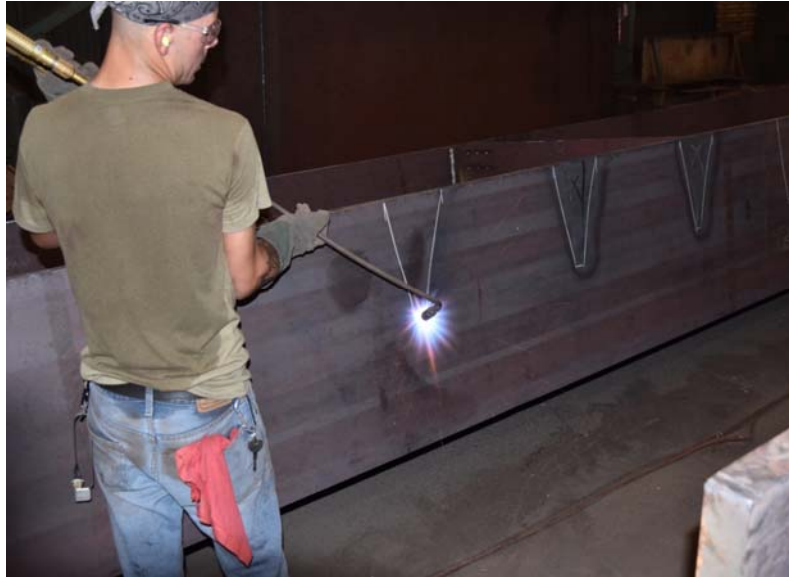
Figure 17: Heat curving of a girder
