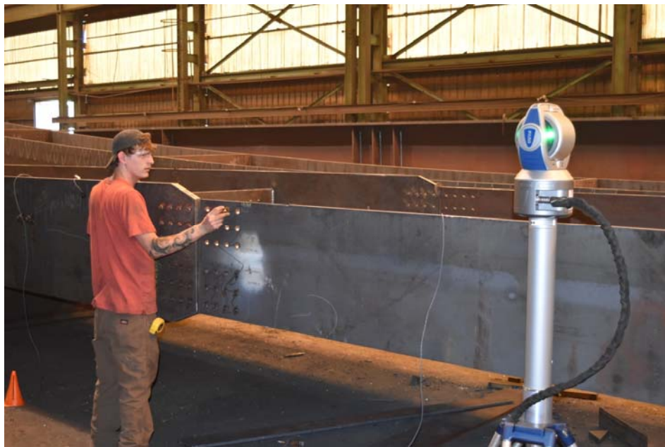
Figure 23: Measuring the locations of the splice connection holes in the girder flange with the laser tracker
