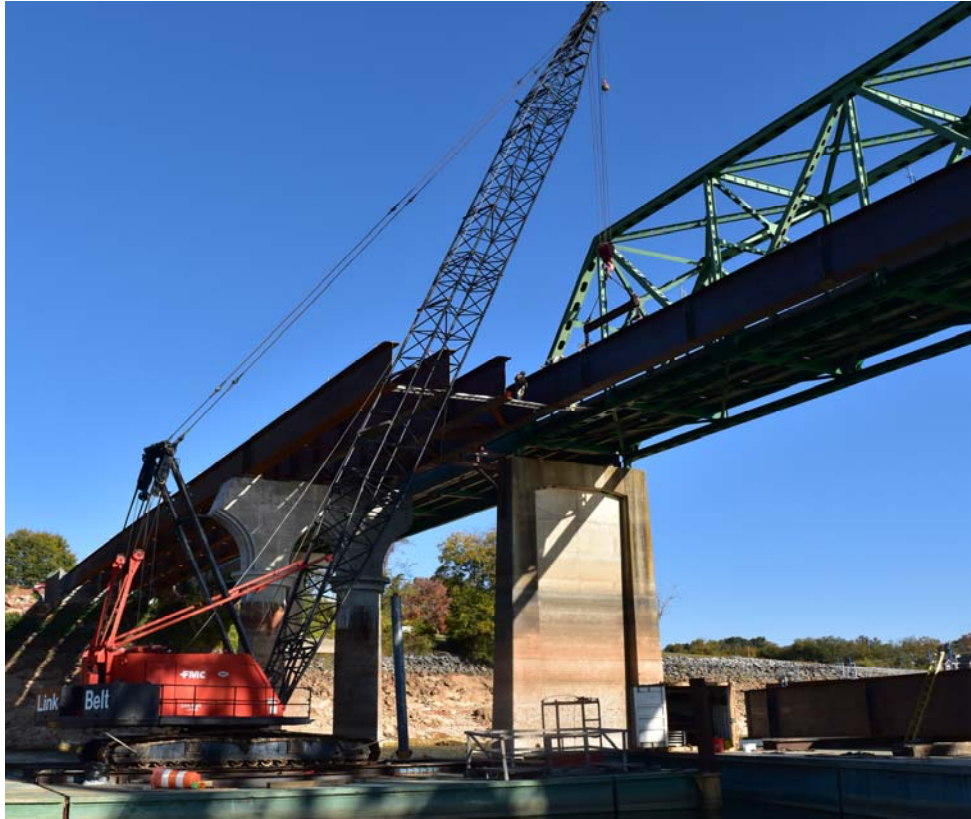
Figure 9: Bottom view of bridges (Older bridge on the right, newer on the left)
