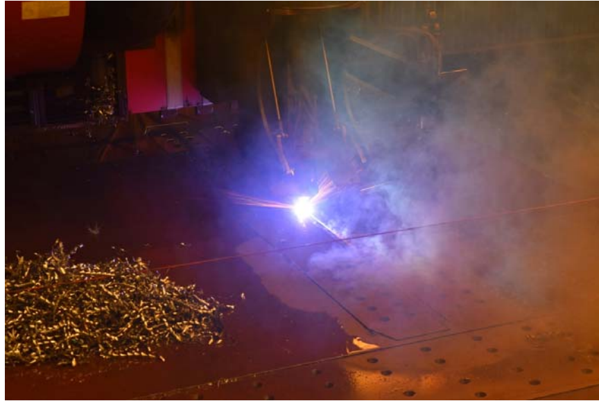
Figure 25: CNC machine plasma cutting a splice plate
