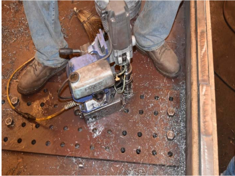
Figure 20: Drilling the web plate (top view). Note the four shop bolts used to hold the plate in place during the drilling process.
