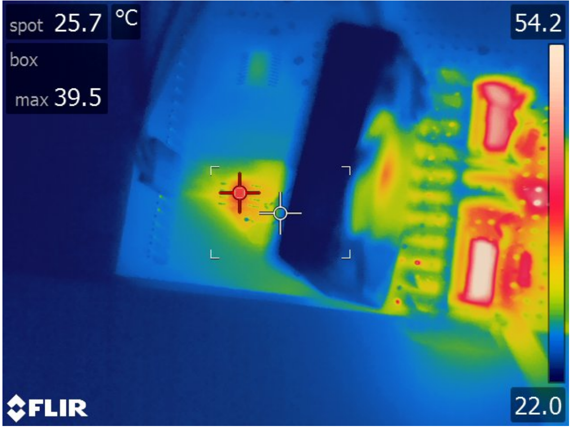
Figure 4.9: Gate Driver Thermal Image from FLIR Camera when P_{out} = 250 W.
