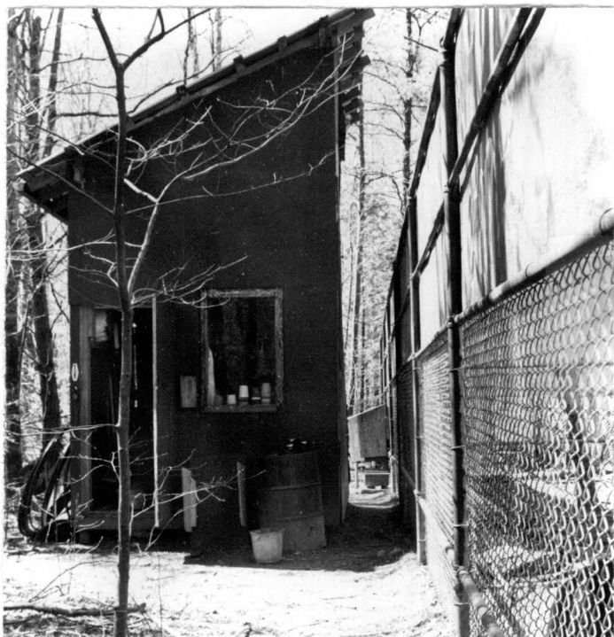
Figure 6. Side view of the observation and storage shed.
