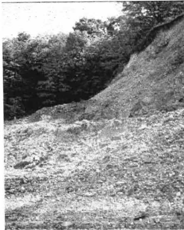
Fig. 7. Steep shale embankment adjacent to gymnasium
