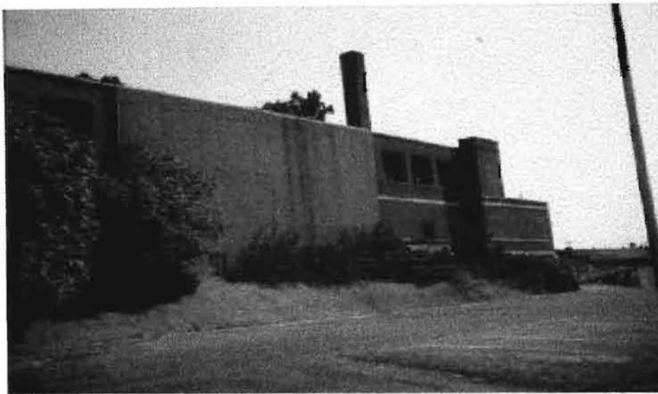
Fig. 6. Gymnasium of the Old Southside Junior High School, view towards SE
