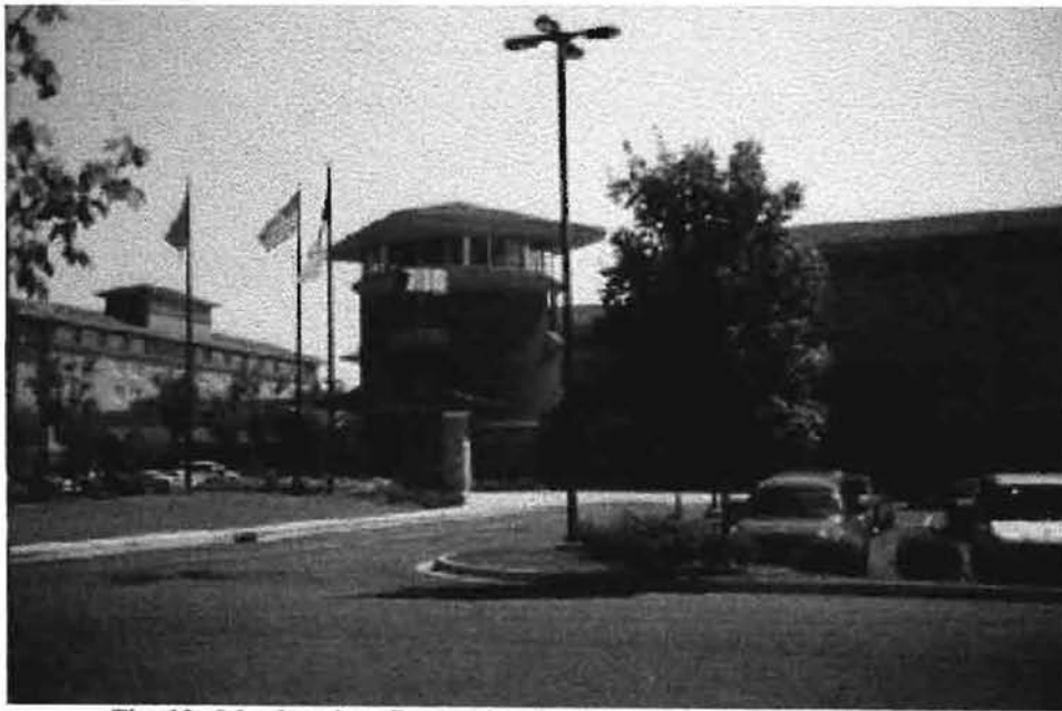
Fig. 12. Meadowview Convention Center and Hotel, main entrance
