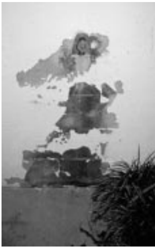
Repair plumbing leaks as quickly as possible. Moisture attracts termites to the structure.
