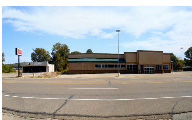
FIG 8. Highway 1 Current conditions in Wynne on Highway 1. (Photo by author)
