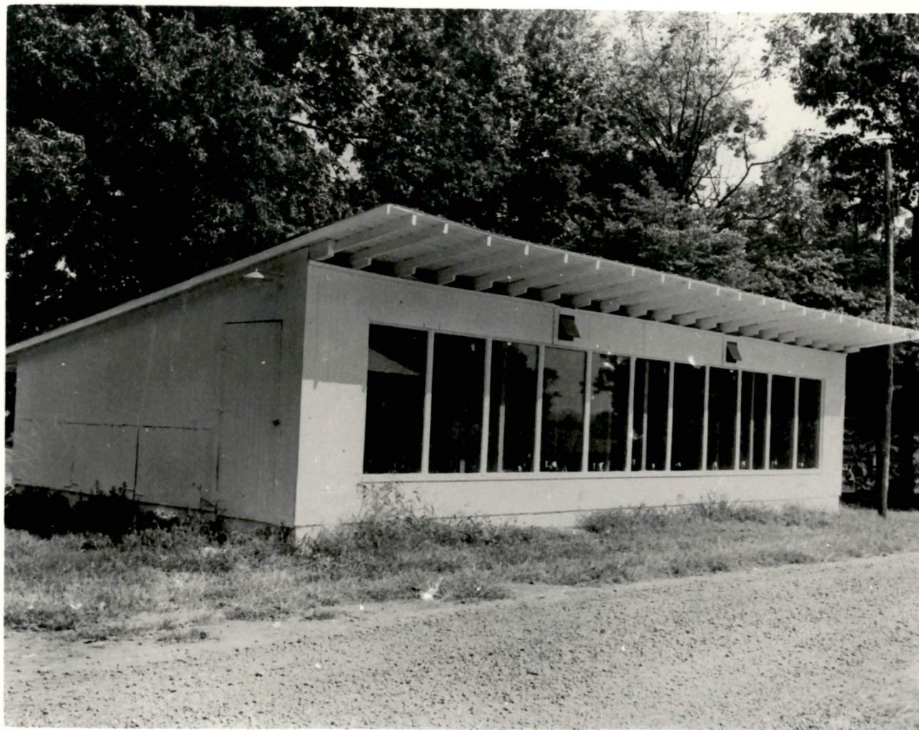
Figure 7. Front view of the Solar House (note ventilation fans).
