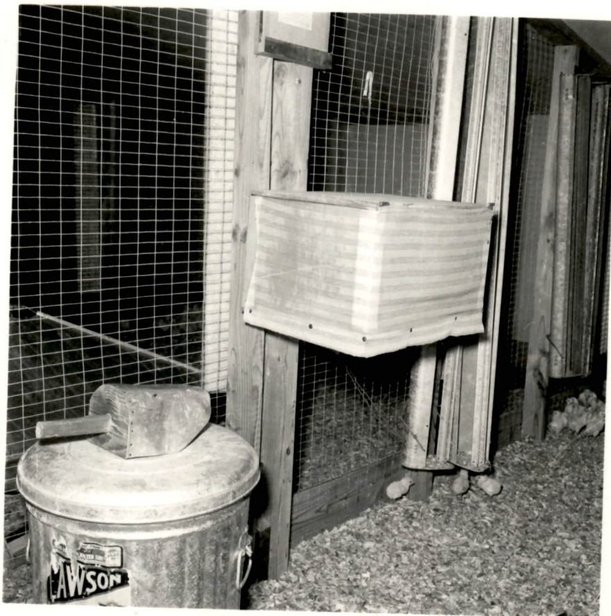
Figure 16. A view of the fan unit filter box mounted inside the house (note the cloth used for filtering purposes).
