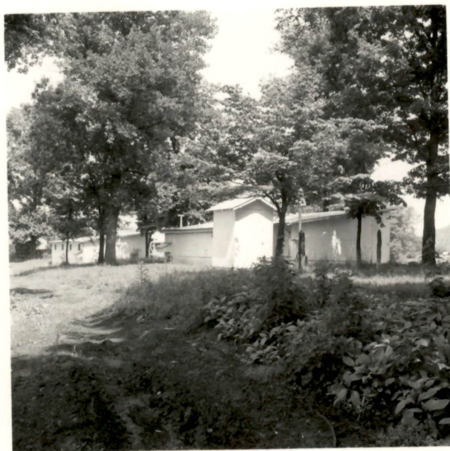
Figure 6. Rear view of the Windowless and Conventional Houses. Also shown is the instrument house.
