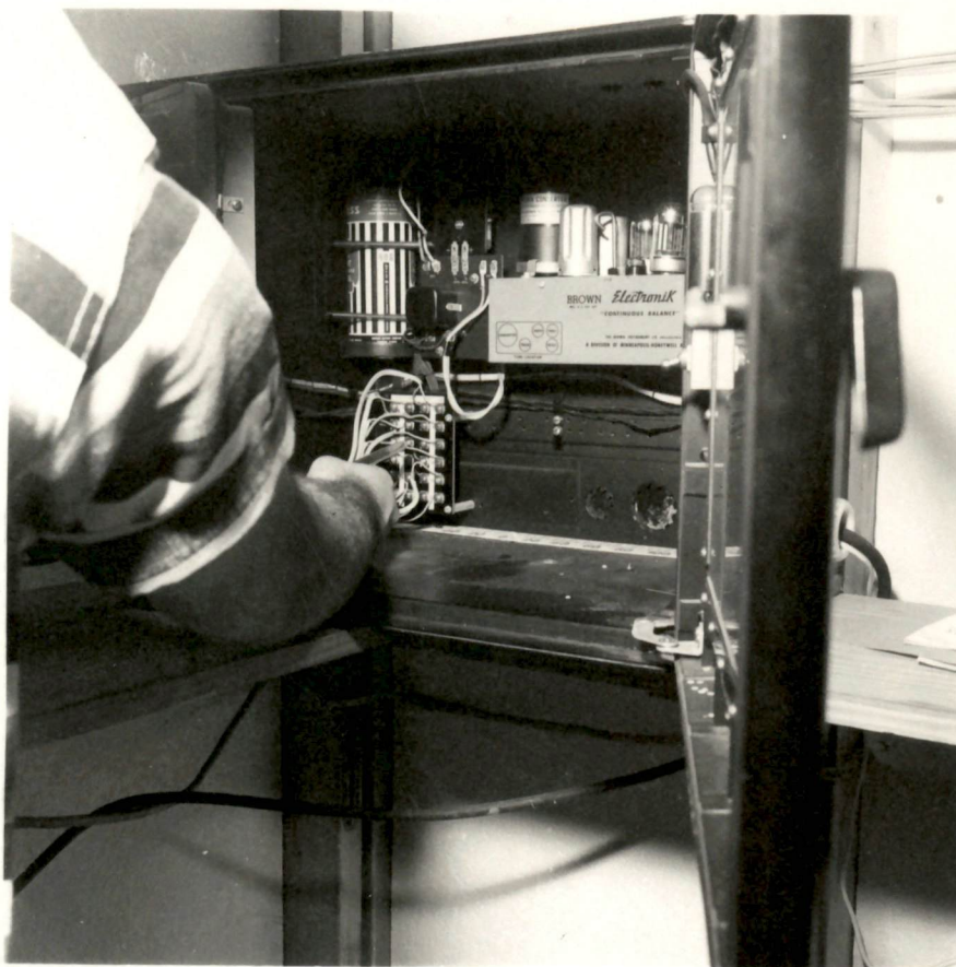
Figure 13. Inside view of the Brown recording potentiometer.
