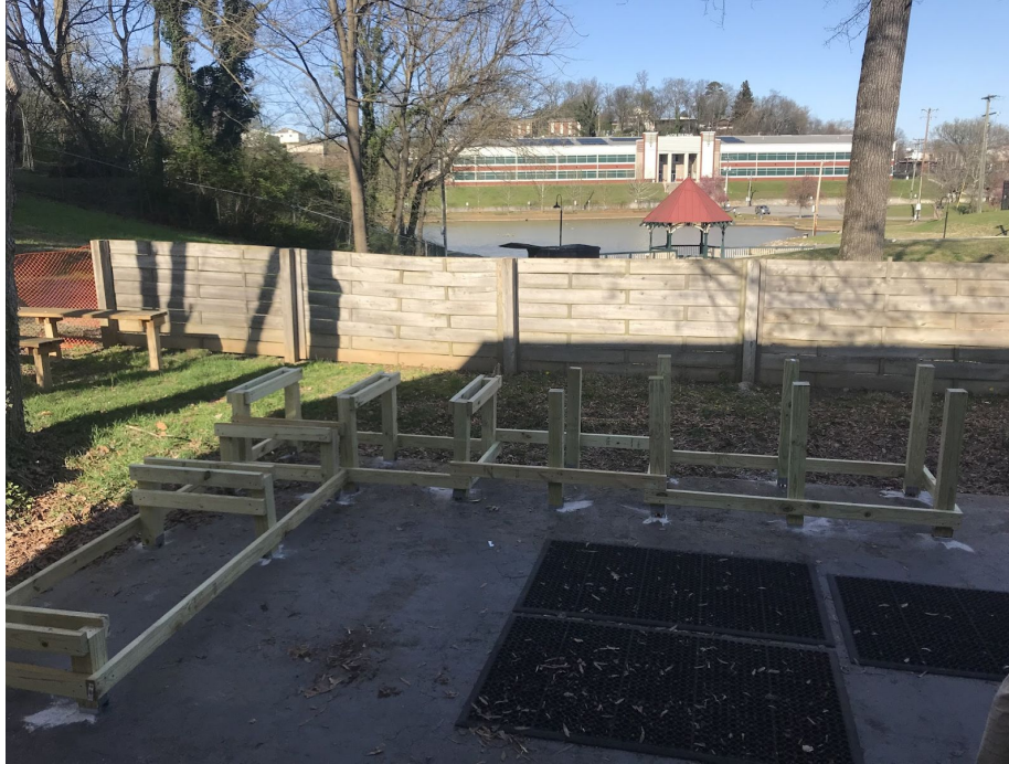
Figure 2. Wood Base Structure
