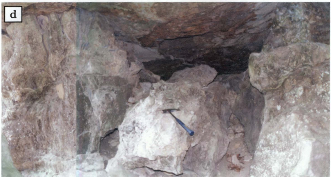
Figure 22 cont. - Photographs of paleo-dolines 3, 4, and 5, and associated features. Figure 22c - The base of paleo-doline 4 has a rounded, but pockmarked appearance. Circled area surrounds a particularly good example of small grooves and pits, which were possibly caused by root growth. Figure 22d - This was once a wall of limestone that separated paleo-dolines 4 and 5. When the wall was breeched, a hole developed that was filled with mantling breccia -conglomerate. Hammer is resting on the fill.
