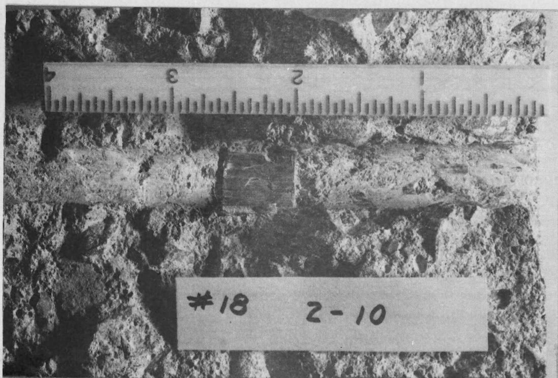
Figure 37. Closeup of 10% air content core containing wedge. Top of core is located to right--Phase I.
