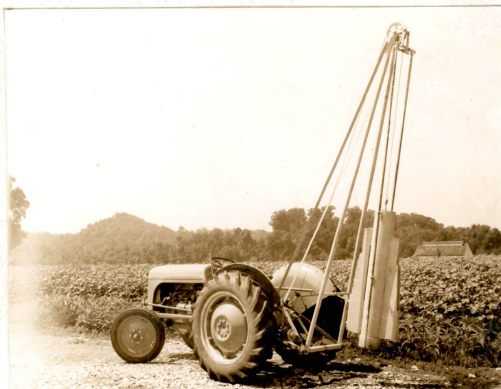
Figure 7 Completed Machine With Driving Head in Transporting Position
