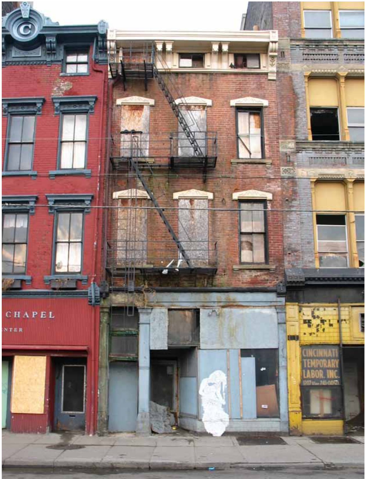
Figure 3: Vacant Building in Over-the-Rhine
