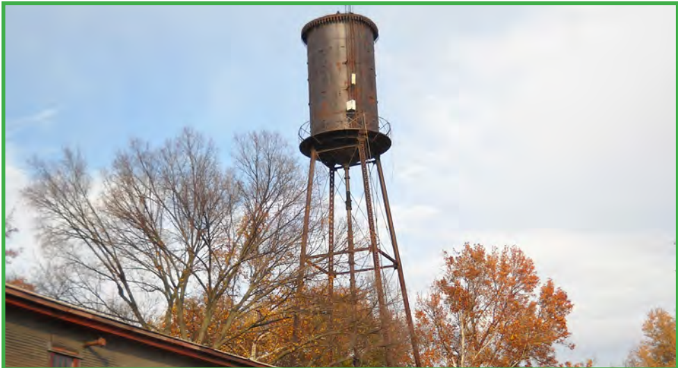
Re-use of Water Tower as Irrigation
