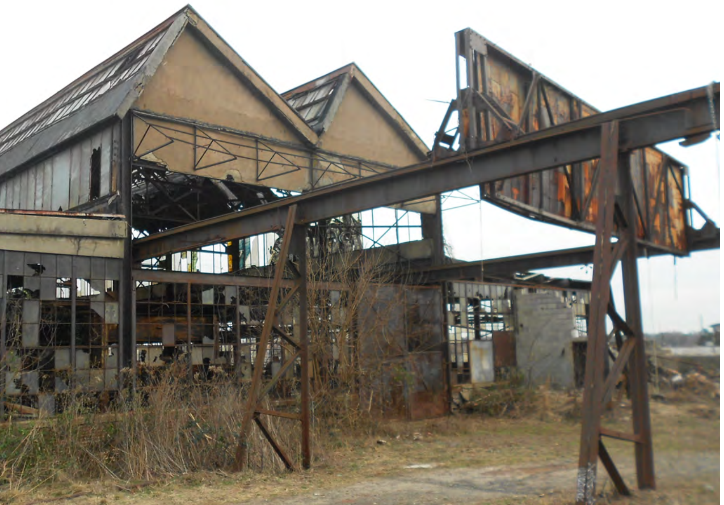
Saw Tooth Roof / Movable Overhead Beam
