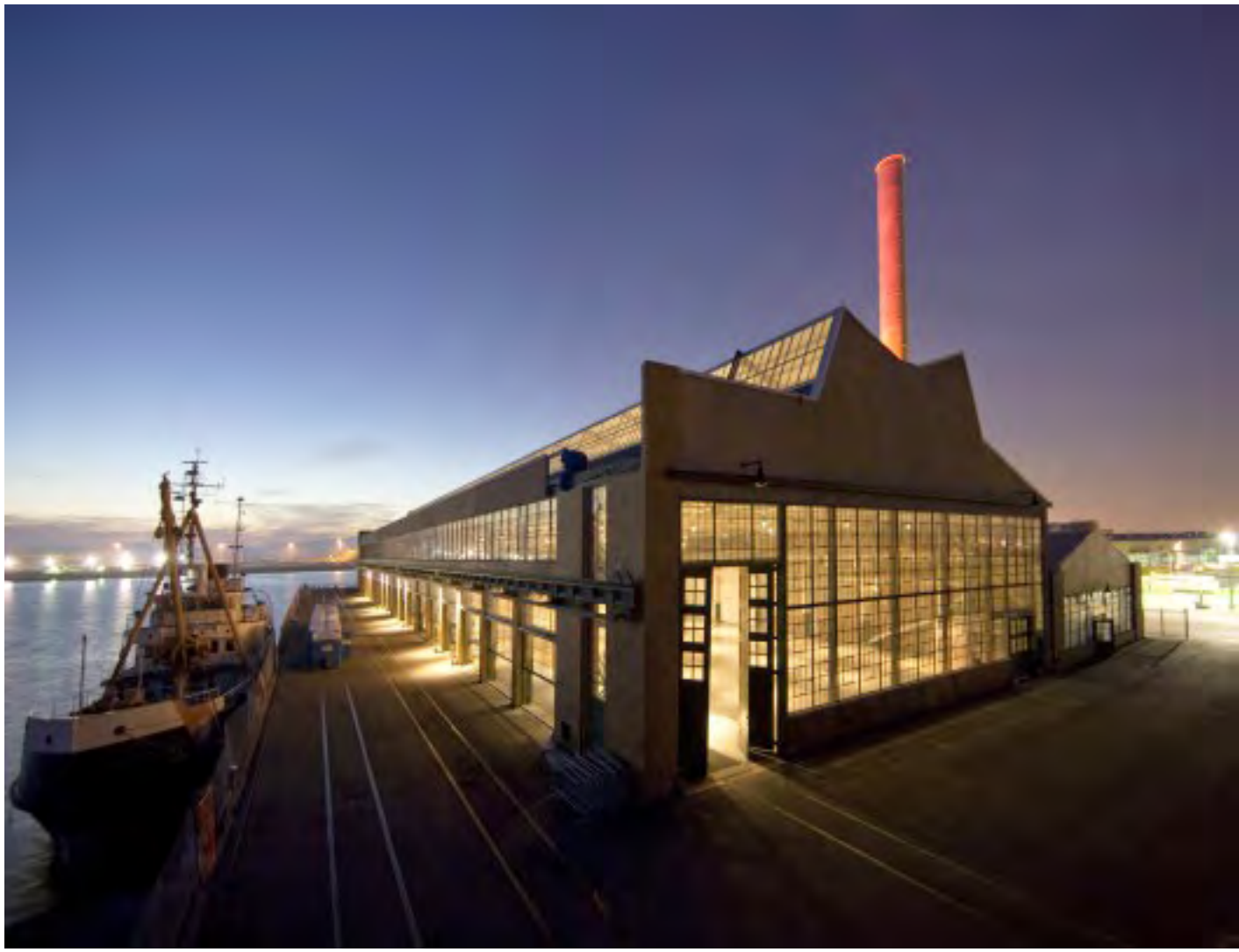
Ford Assembly Building
