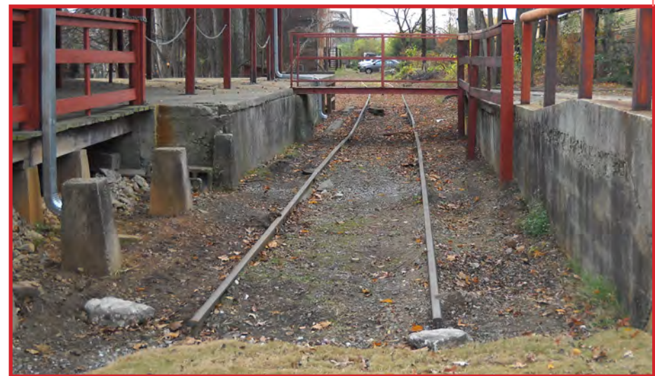
Historical Railroad Tracks
