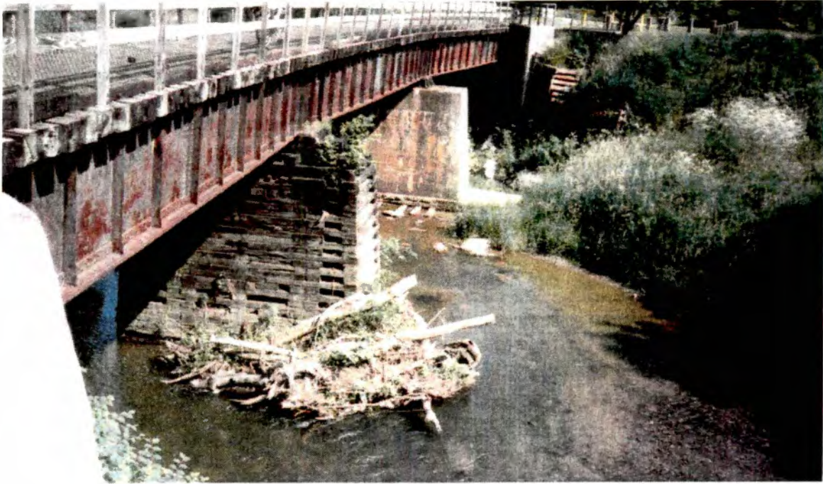
Figure 1. Woody debris accumulation at a bridge pier along the New River Trail in southwest Virginia. (Photo courtesy of Tschantz)
