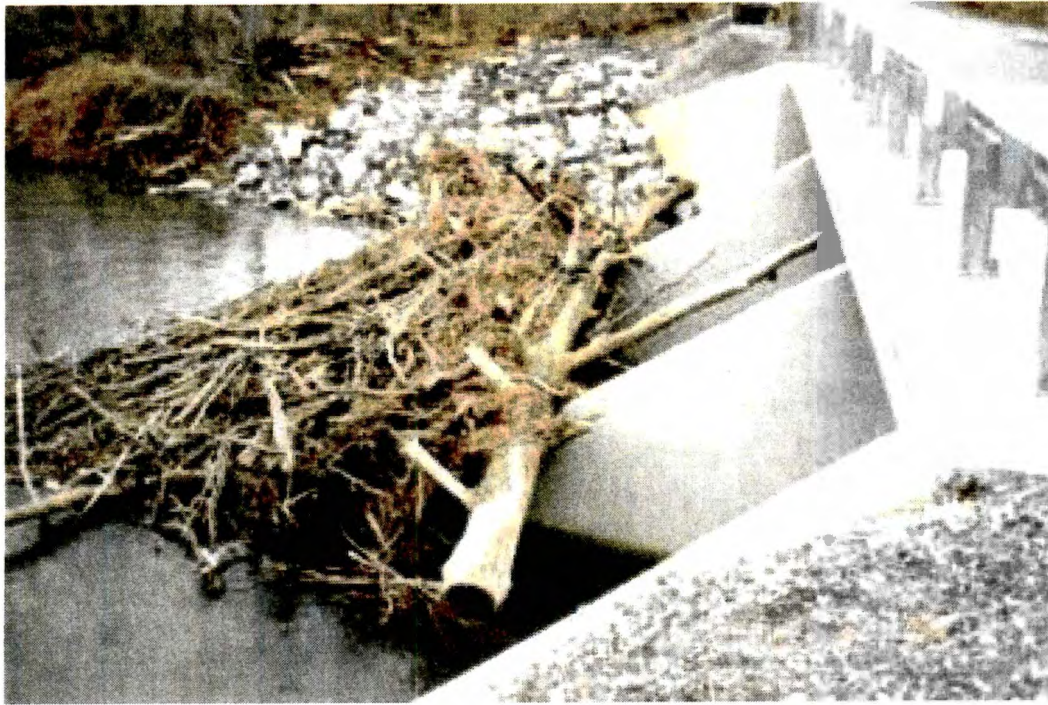
Figure 5. Debris fins with drift accumulation. (from Tennessee Department of Transportation, 1998)
