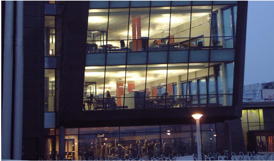
Figure 192. Telenor office building. Photo Jan Draplos
