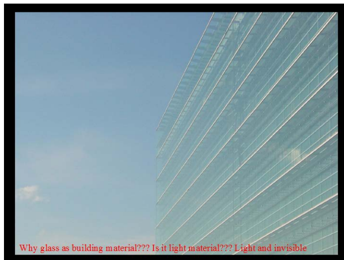
Figure 156. Invisible façade of building. Photo Vesa Honkonen
