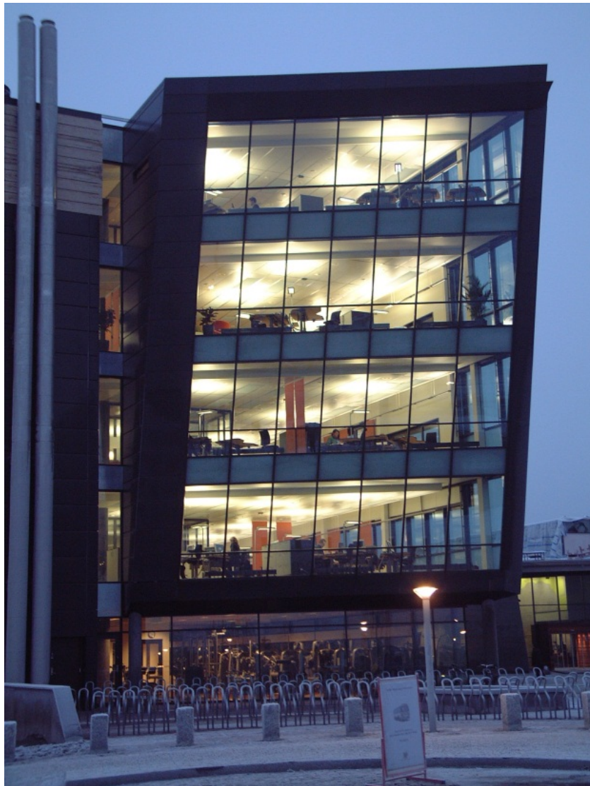
Figure 191. Telenor office building. Photo Jan Draplos
