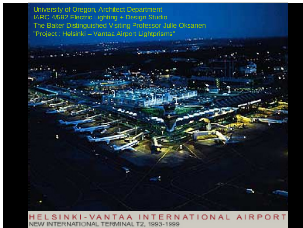
Figure 206. Helsinki - Vantaa airport. Photo Finavia
