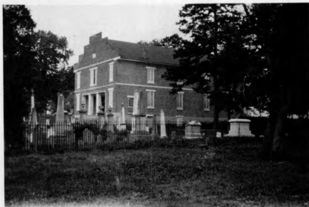
ZION Presbyterian Church and Church Yard.
