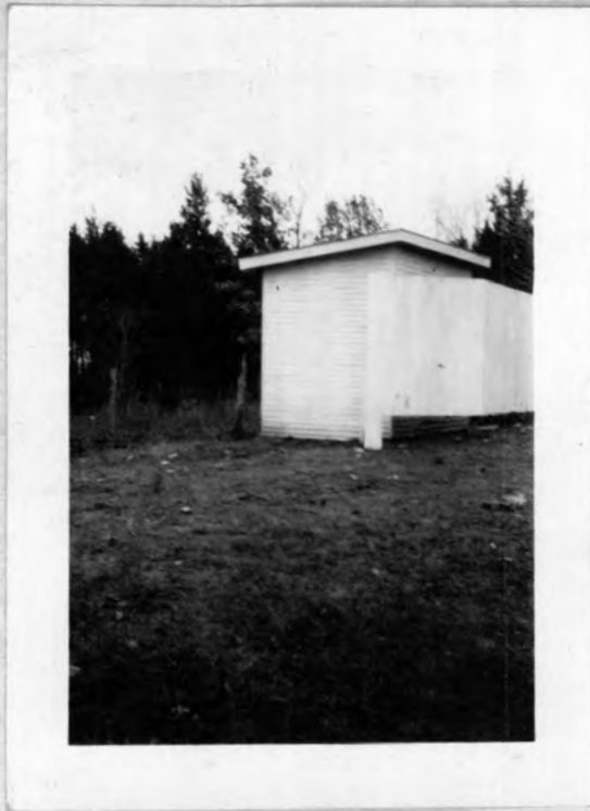
NEW SANITARY TOILET. UNION GROVE.
