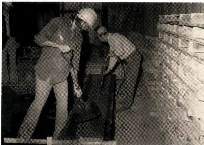
(a) Placement and compaction of concrete
