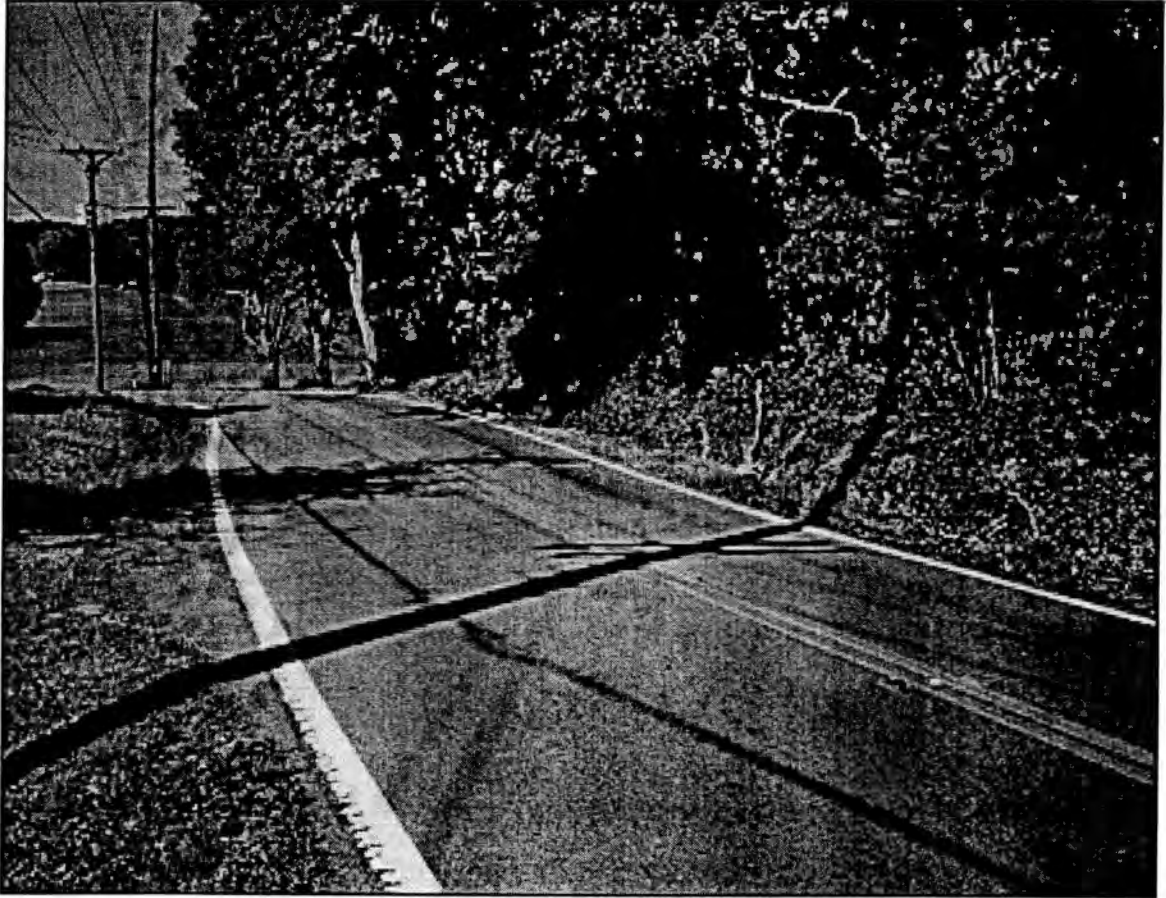
Figure 9. Horizontal curvature at the E. Emory Rd. site.
