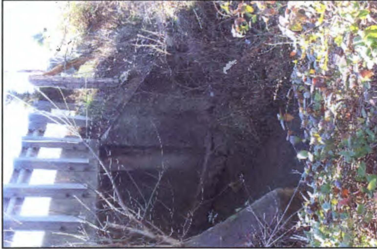
C. An exposed bridge footing at TS01.
