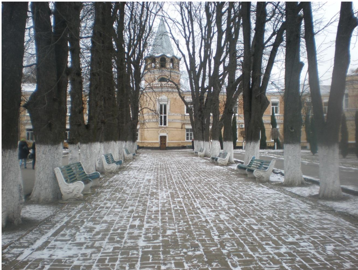
Figure 1 Administrative Building of state-run Psychiatric Hospital in South Central Ukraine
