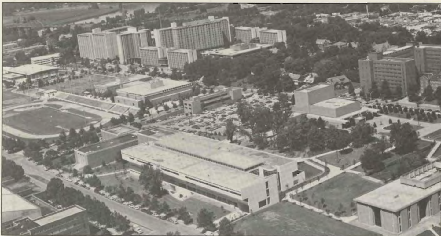
The Art-Architecture Building, lower center, was completed during the year. Occupancy of the Knoxville campus building occurred this summer. At left is an interior view of the building.
