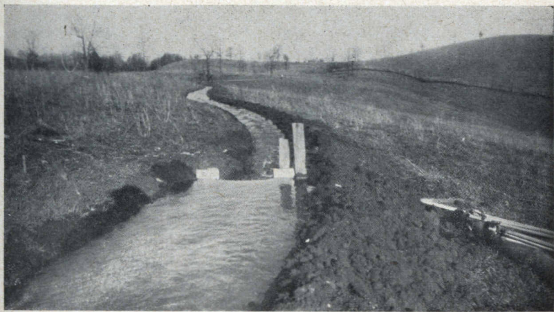
Fig. 39—An experimental irrigation ditch.
