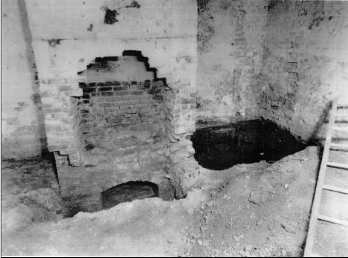
Figure 3.7. Milton Grigg's 1941 exploratory excavation photo of the northwestern portion of the South Pavilion (O'Connor and Neiman 2022:37).
