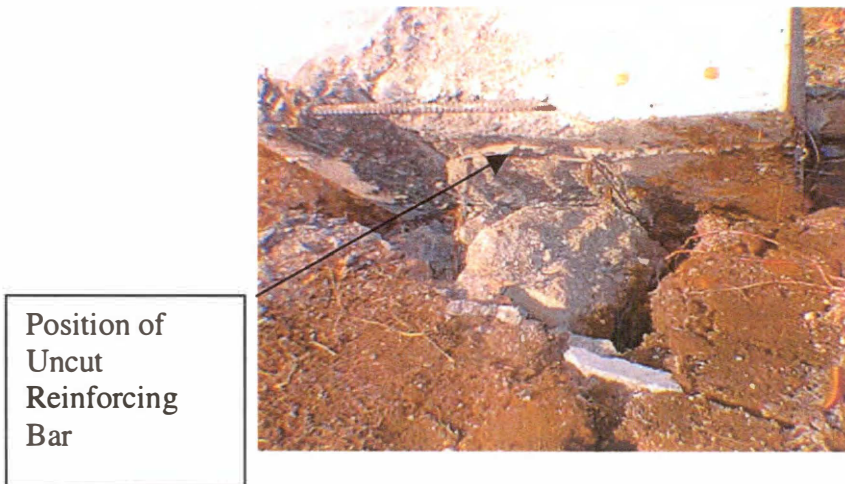
Figure A7.9: Pile 2 Interface 2
