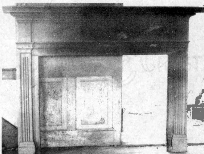
Figure 37. Boyd House: Mantel.
