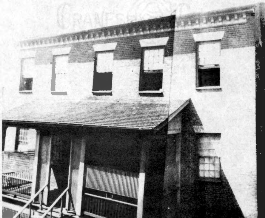
Figure 29. Park Mansion: Facade.
