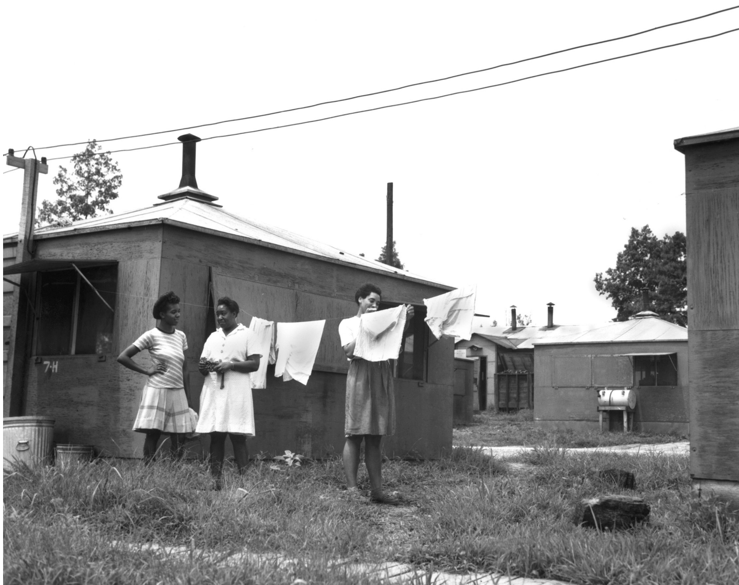
Civil Engineering Works Housing: African-American Hutments, August 10, 1945
