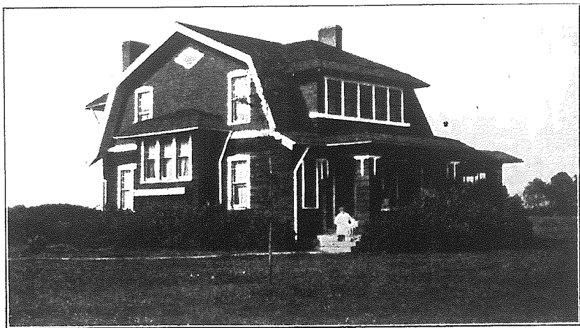
SUPERINTENDENT'S RESIDENCE WEST TENNESSEE EXPERIMENT STATION, JACKSON
