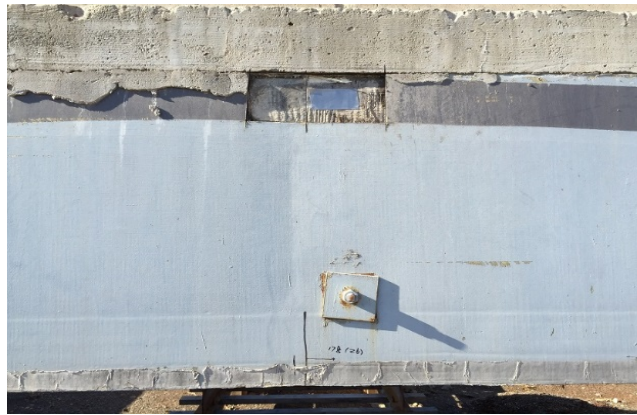
Figure 3.10 Small Window Cutout of FRP Shell
