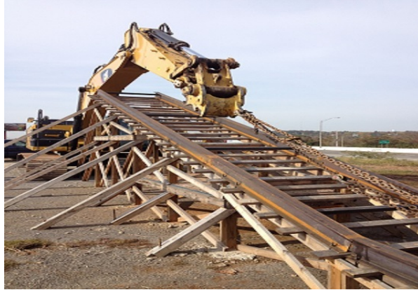
Figure 2.3 Track System and Excavator
