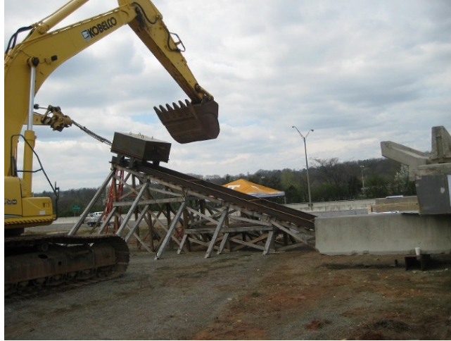
Figure 3.12 Impact Cart and Second Excavator
