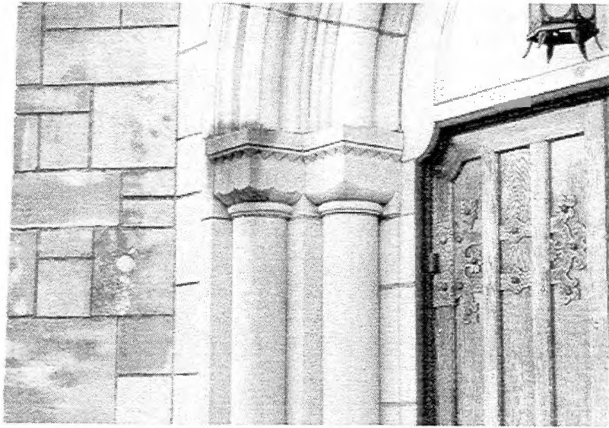
Figure 20: Detail of column capital, Holy Ghost Church, Knoxville, Tennessee
