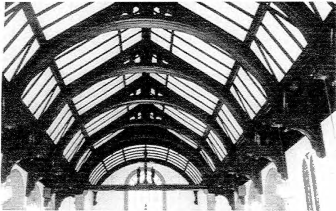
Figure 81: Ceiling, Holy Ghost Church, Knoxville, Tennessee
