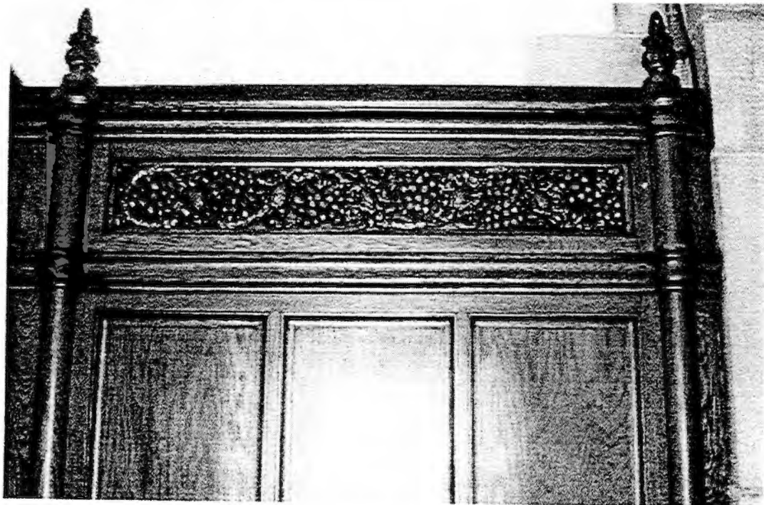
Figure 57: Panel detail, Holy Ghost Church, Knoxville, Tennessee
