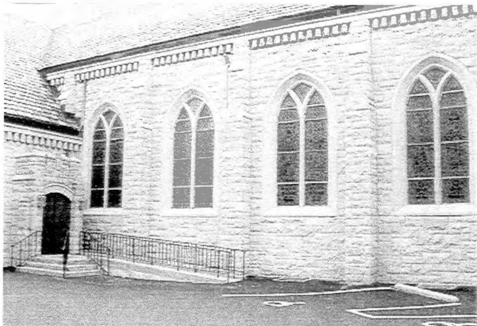
Figure 16: Buttresses and corbel-table on north elevation, St. Catherine Church, Cincinnati, Ohio
