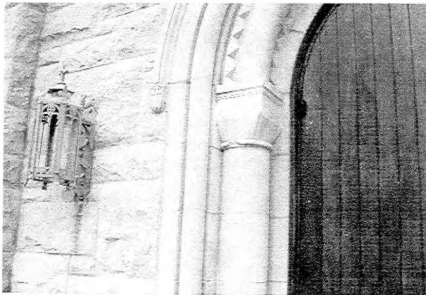
Figure 21: Detail of Column Capital, St. Catherine Church, Cincinnati, Ohio
