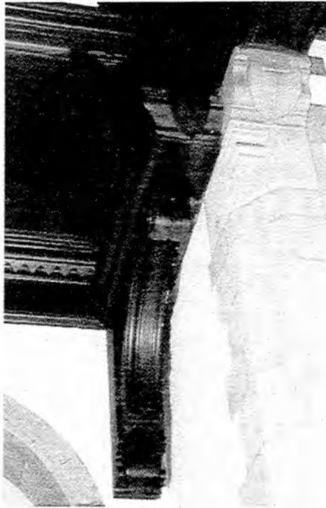
Figure 82: Ceiling detail, Holy Ghost Church, Knoxville, Tennessee
