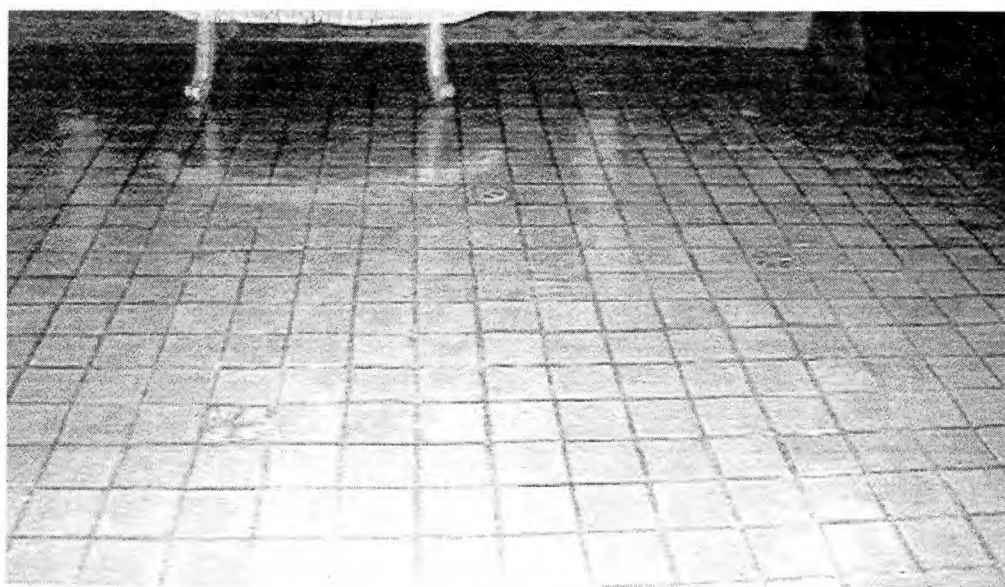
Figure 80: Floor tiles, Holy Ghost Church, Knoxville, Tennessee
