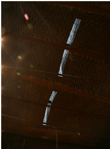
Figure 28: Apertures in Vaulted Roof Source: Ted Shelton
