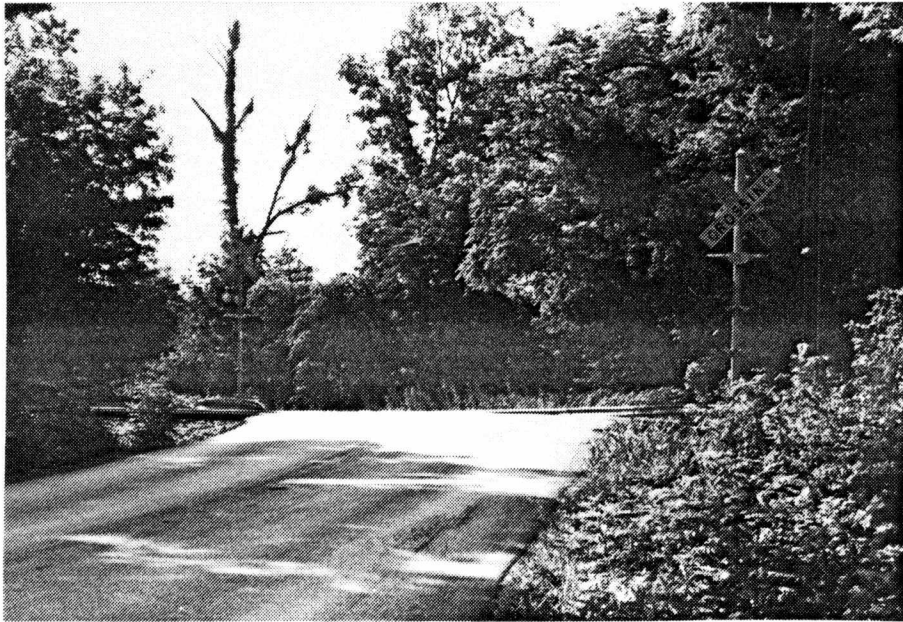
Figure 29. Ebenezer Road crossing--flashing light signals.
