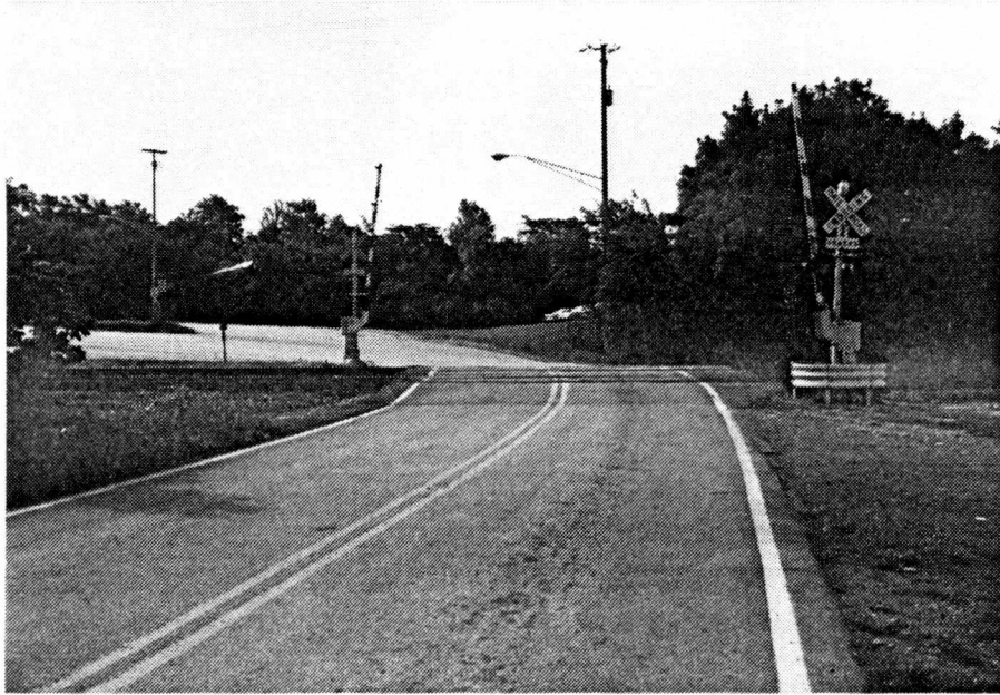
Figure 30. Prosser Road crossing--gates with flashing light signals.
