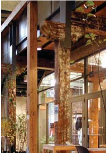
Fig. 14 Interior of the Ecotrust Building Source: dominekarch.com
