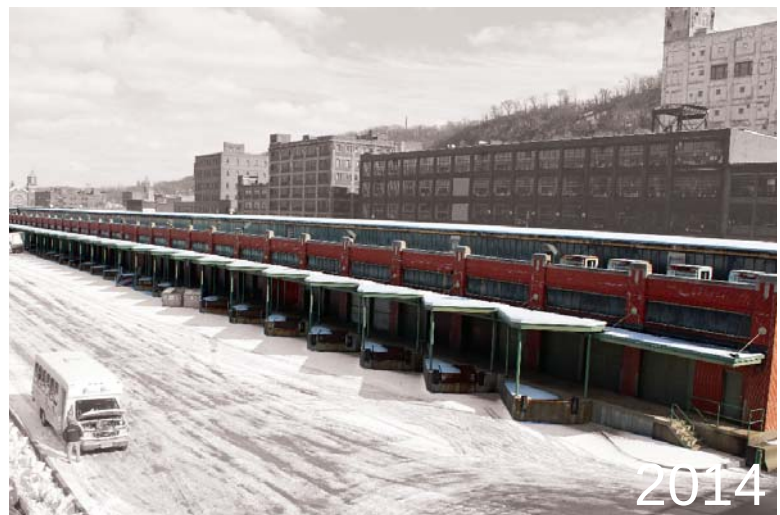
Fig. 32 Existing Conditions, Loading Docks Source: author
