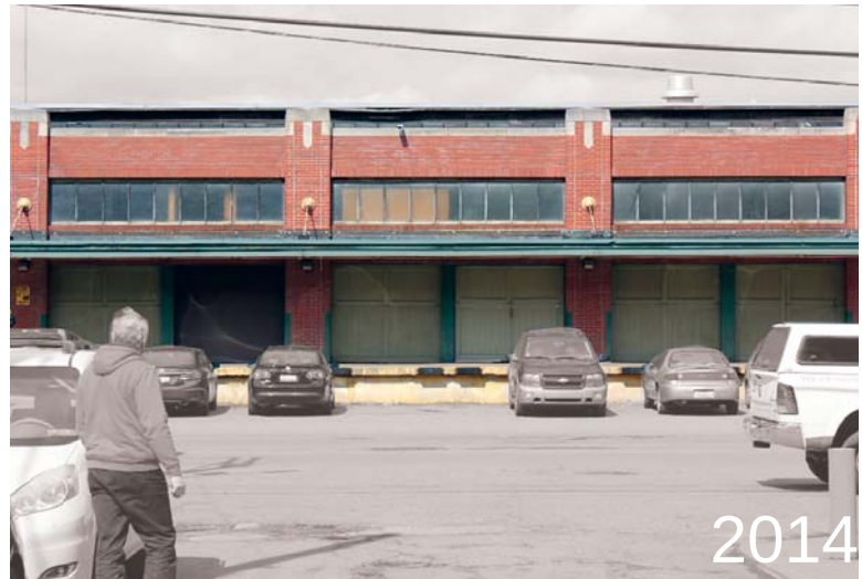
Fig. 31 Existing Conditions, Smallman Street Source: author
