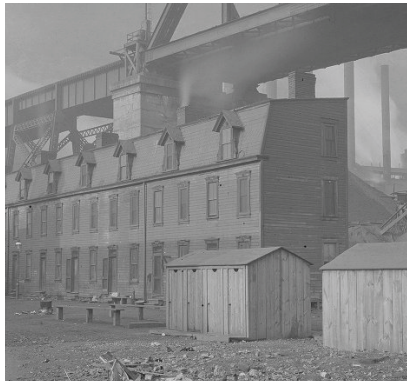
Fig. 02 - Worker Housing Source: Pittsburgh & Lake Erie RR Company Photographs
