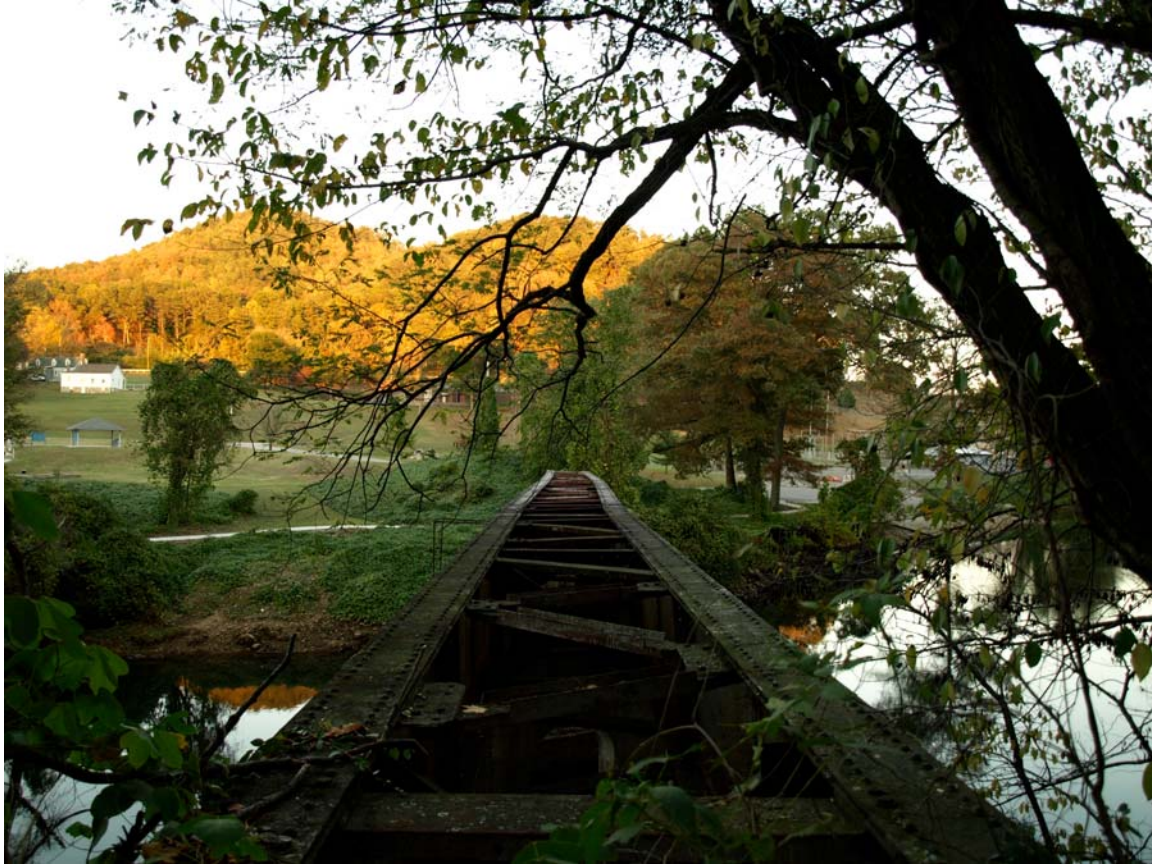
Figure 24 a: The existing abandoned TVA railroad bridge is a great opportunity to rehabilitate to provide pedestrian and bicycle access across the Ocoee River. Source: Nathan Oliver
