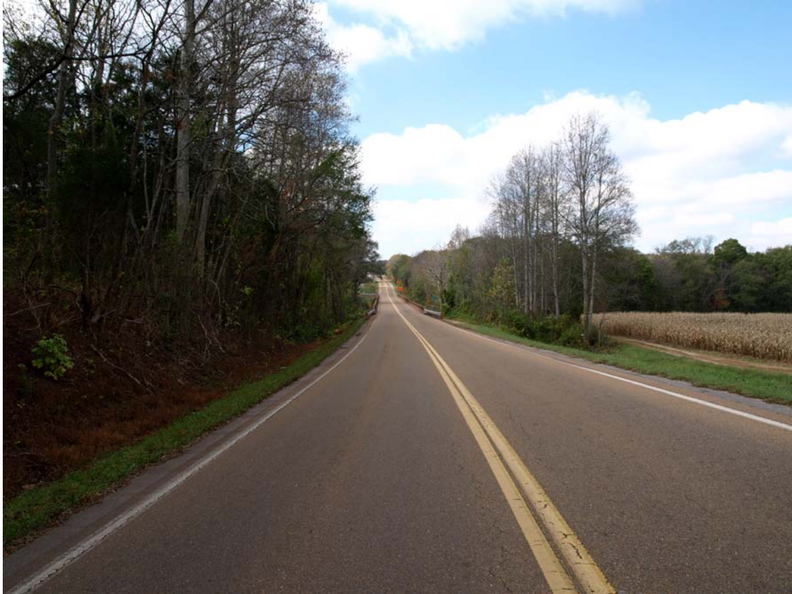
Figure 10: View of existing Highway 64 in Parksville at the project boundary and existing construction of Corridor K. Source: Nathan Oliver
