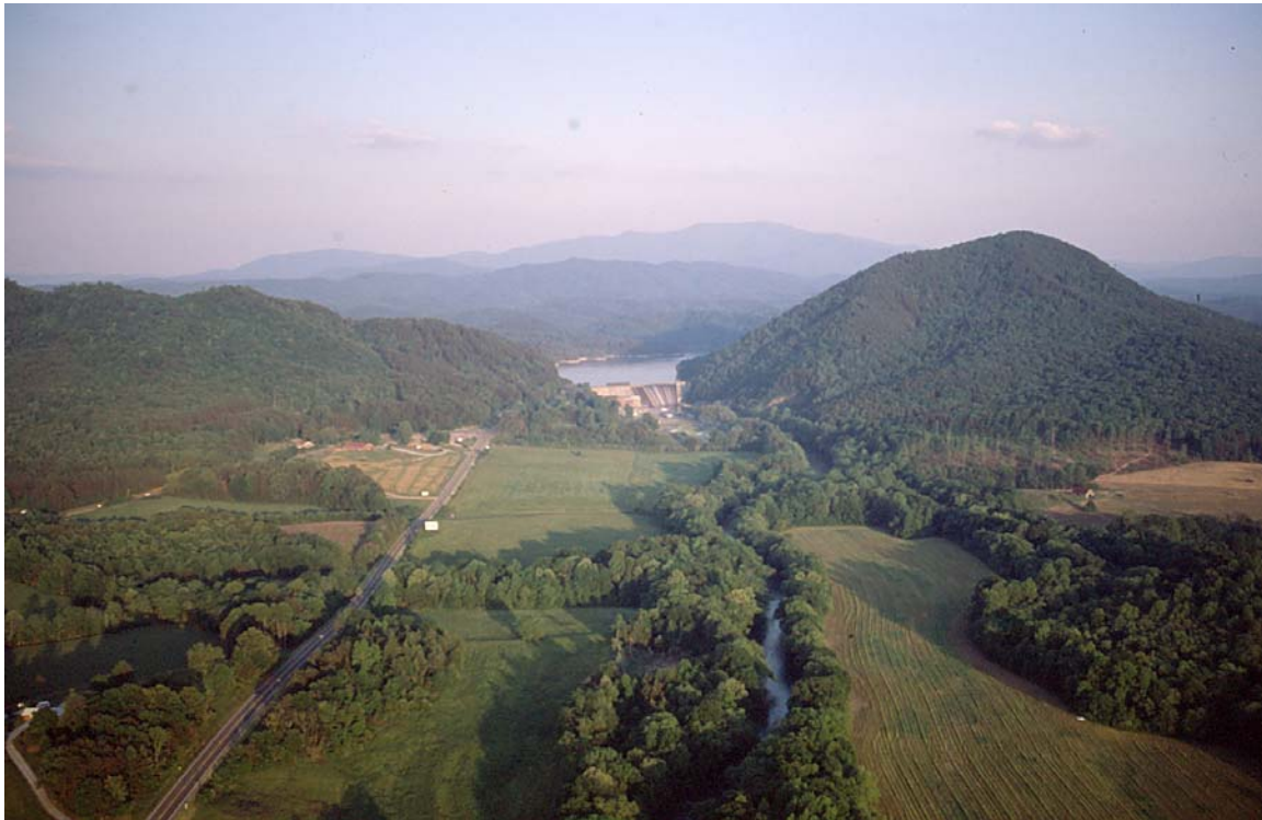
Figure 7: View of the terrain and landscape of Parksville and the surrounding area. Source: Sam Rogers
