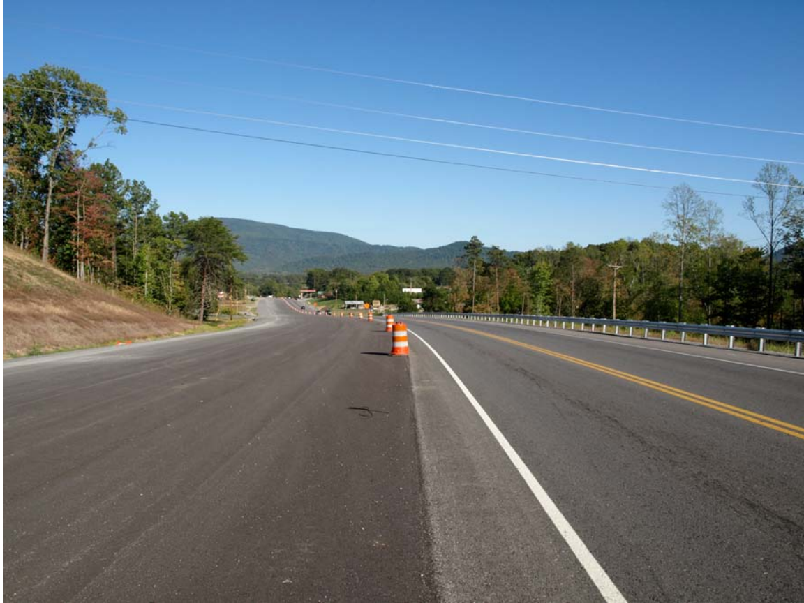
Figure 9: View of existing construction of Corridor K before entering the project area. (Typical 5-lane, 2-shoulder design) Source: Nathan Oliver
