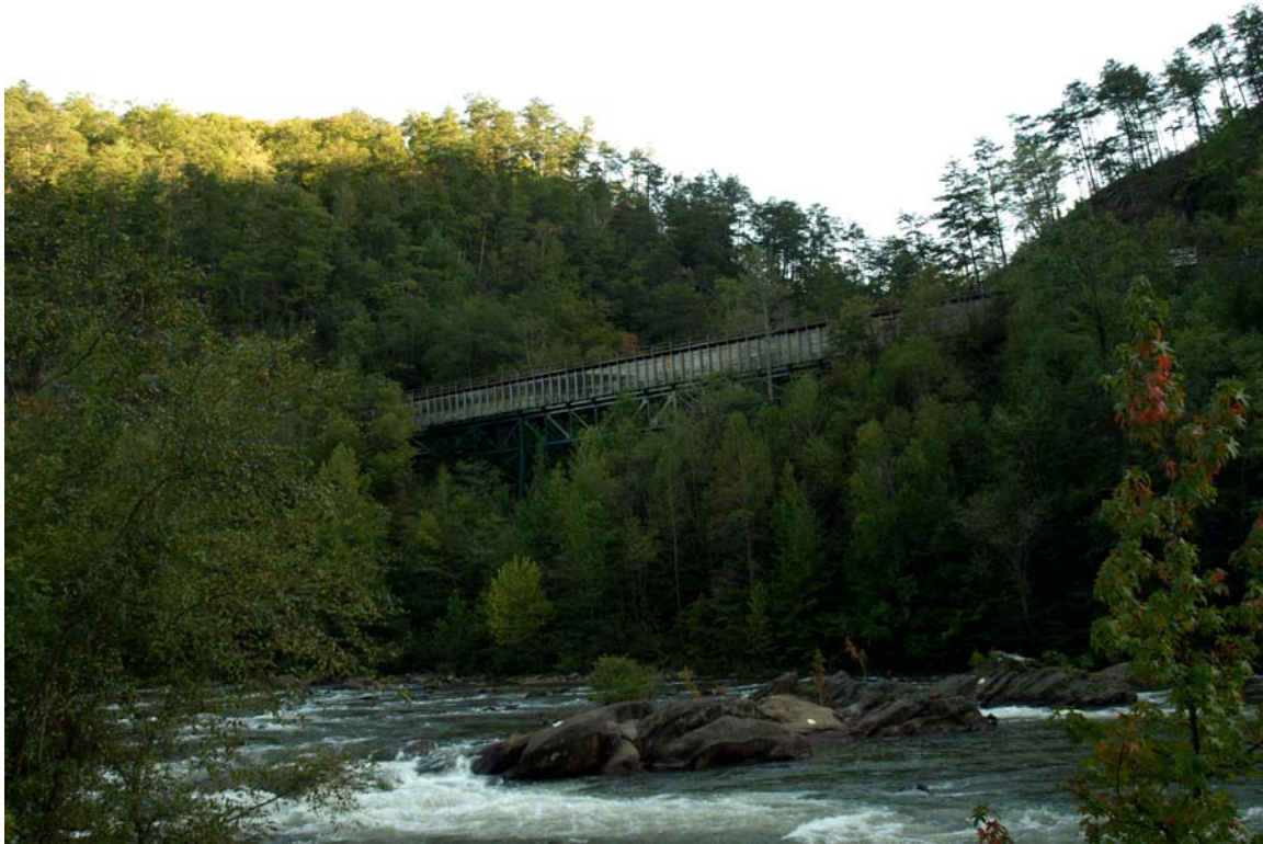
Figure 18: A section of the wooden flume between Dam #2 and the powerhouse, and still functioning today. Source: Nathan Oliver
