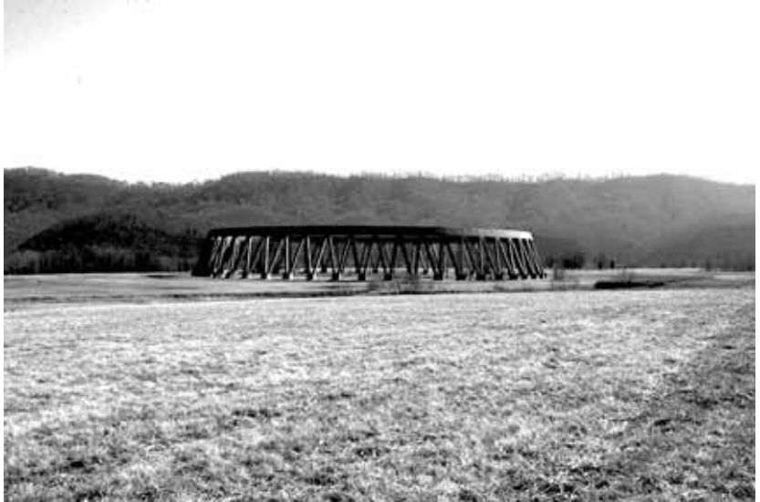
figure_27. View of cooling tower base as approached on axis from southeast edge of Phipp's Bend Industrial Park (diagram describing axis of movement and cone of vision). SOURCE: author.
