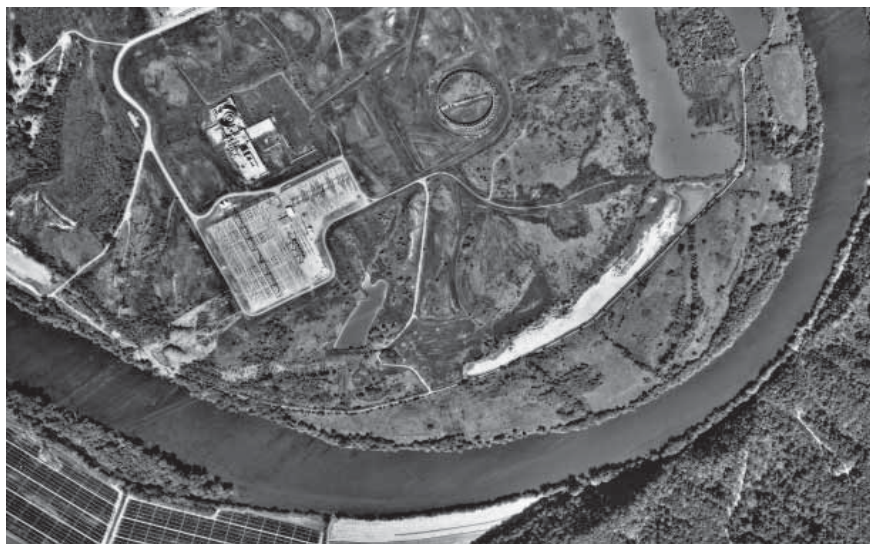
figure_21. Aerial image of site. Phipp's Bend Industrial Park near Surgoinsville, Tennessee. Focused on abandoned nuclear reactor facility. SOURCE: Professor T. K. Davis
