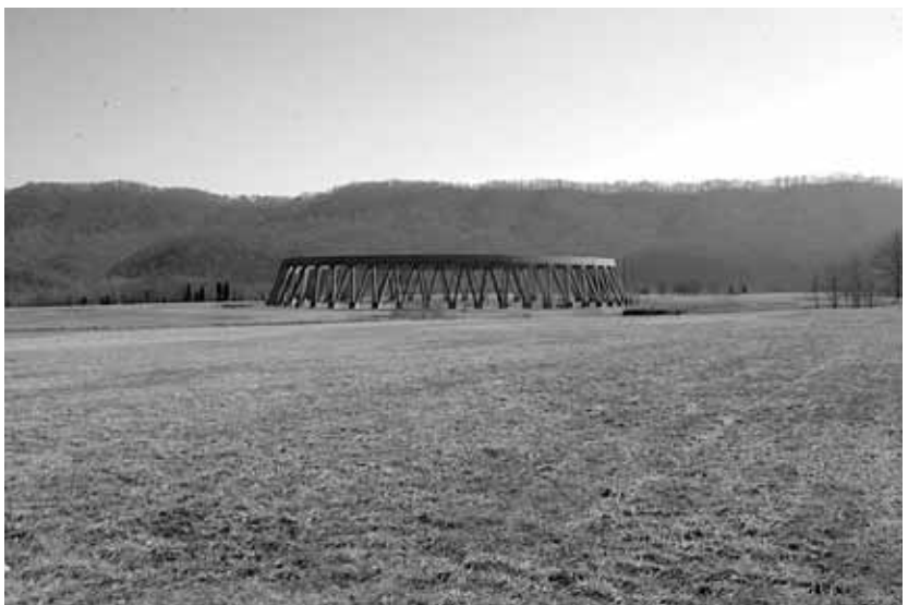
figure_26. View of cooling tower base as approached on axis from southeast edge of Phipp's Bend Industrial Park (diagram describing axis of movement and cone of vision). SOURCE: author.
