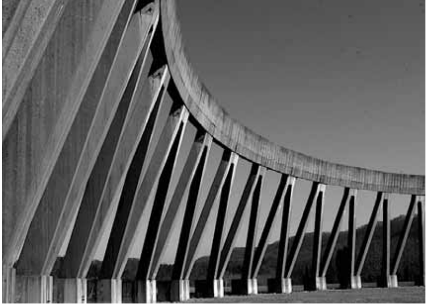
figure_36. View of cooling tower base looking west from directly below beam as approached from southeast edge of Phipp's Bend Industrial Park (diagram describing axis of movement and cone of vision). SOURCE: author.
