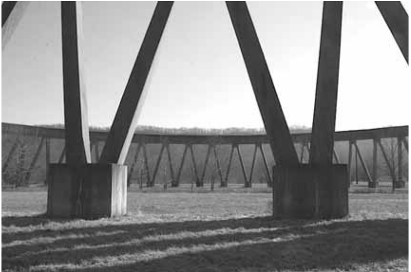
figure_32. View of cooling tower base as approached on axis from southeast edge of Phipp's Bend Industrial Park (diagram describing axis of movement and cone of vision). SOURCE: author.
