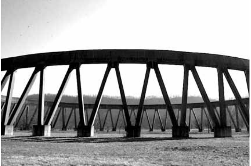
figure_31. View of cooling tower base as approached on axis from southeast edge of Phipp's Bend Industrial Park (diagram describing axis of movement and cone of vision). SOURCE: author.
