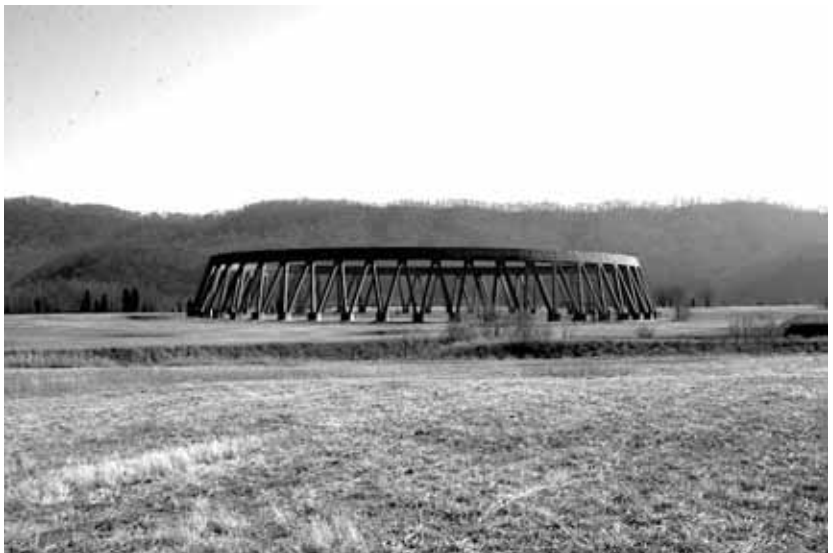
figure_28. View of cooling tower base as approached on axis from southeast edge of Phipp's Bend Industrial Park (diagram describing axis of movement and cone of vision). SOURCE: author.
