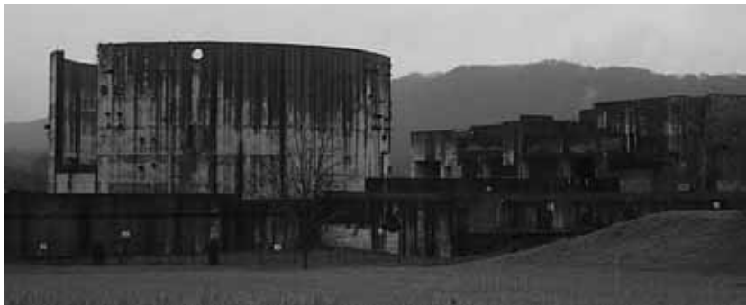
figure_46. View of reactor core housing from northwest corner of site looking southwest. SOURCE: Professor T. K. Davis
