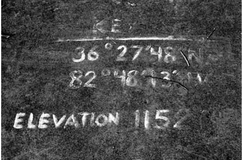
figure_43. Handpainted "key" marking latitude, longitude, and elevation at center of cooling tower base. SOURCE: author.
