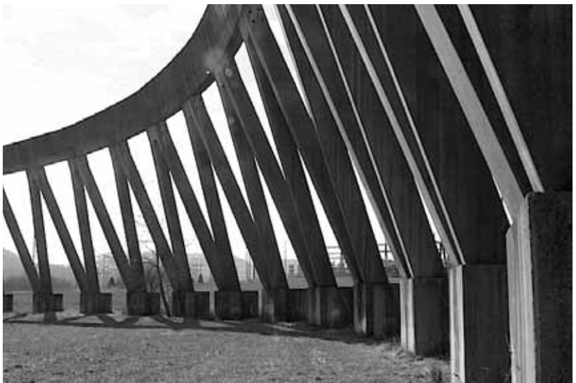
figure_35. View of cooling tower base looking east from directly below beam as approached from southeast edge of Phipp's Bend Industrial Park (diagram describing axis of movement and cone of vision). SOURCE: author.
