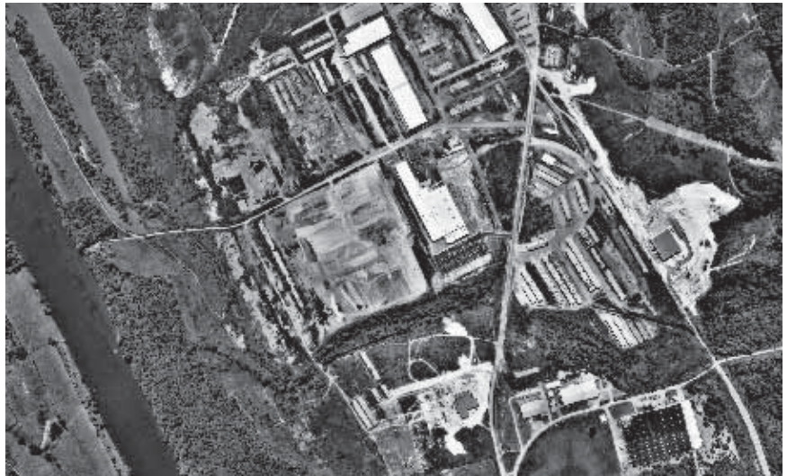
figure_20. Aerial image of site. Phipp's Bend Industrial Park near Surgoinsville, Tennessee. focused on abandoned nuclear reactor facility. SOURCE: Professor T. K. Davis.
