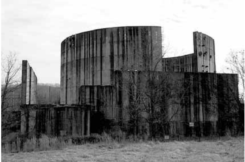
figure_45. View of unfinished reactor building X-21 at Phipp's Bend looking east-southeast. TVA transfer station visible in background. SOURCE: author.
