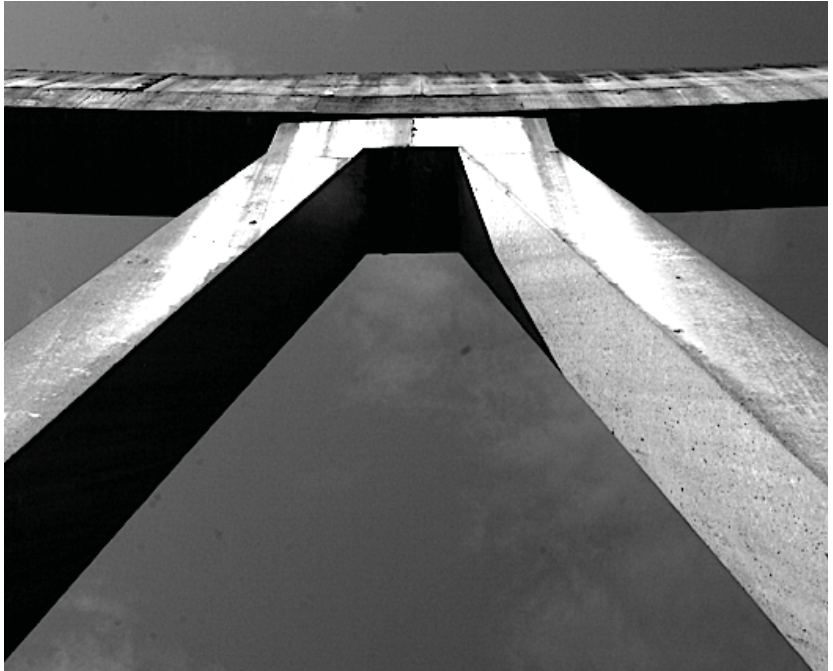
figure_34. View immediately inside threshold of cooling tower base looking skyward as approached from southeast edge of Phipp's Bend Industrial Park (diagram describing axis of movement and cone of vision). SOURCE: author.
