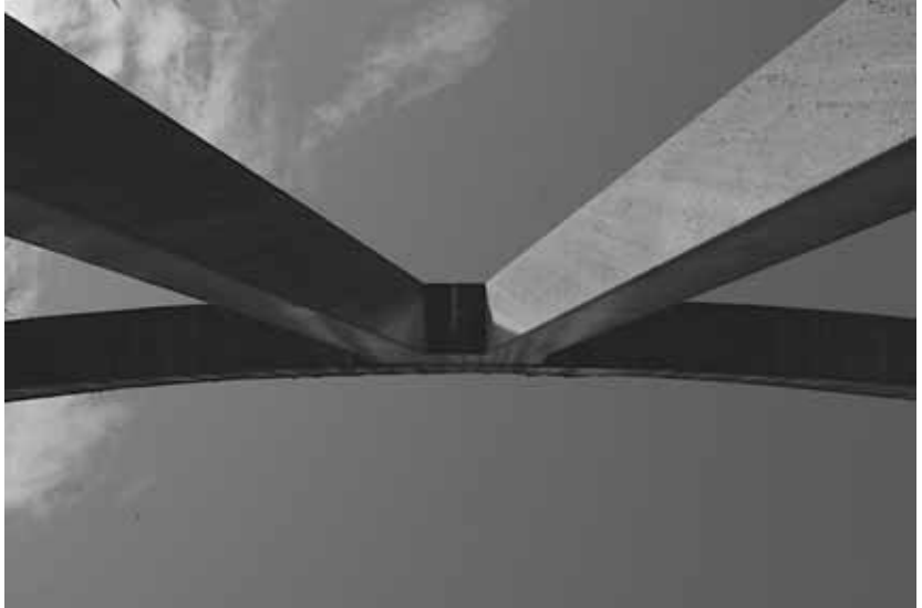
figure_33. View crossing threshold of cooling tower base looking skyward as approached from southeast edge of Phipp's Bend Industrial Park (diagram describing axis of movement and cone of vision). SOURCE: author.
