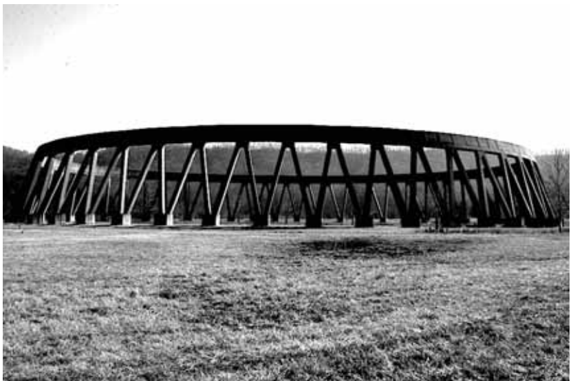
figure_30. View of cooling tower base as approached on axis from southeast edge of Phipp's Bend Industrial Park (diagram describing axis of movement and cone of vision). SOURCE: author.
