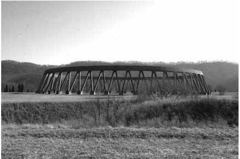
figure_29. View of cooling tower base as approached on axis from southeast edge of Phipp's Bend Industrial Park (diagram describing axis of movement and cone of vision). SOURCE: author.
