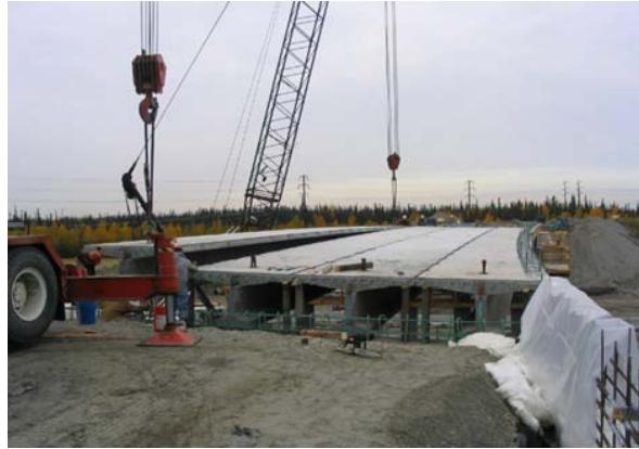
Fig. 4.1. A DBT concrete bridge being constructed
