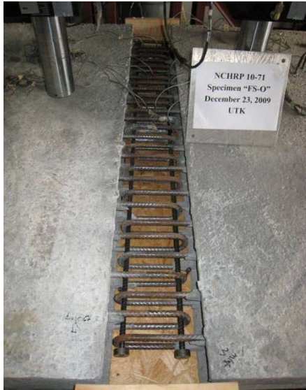
(a) Before grouting
