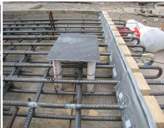
(b) Foam wedges and Pipes Fixed in Place
