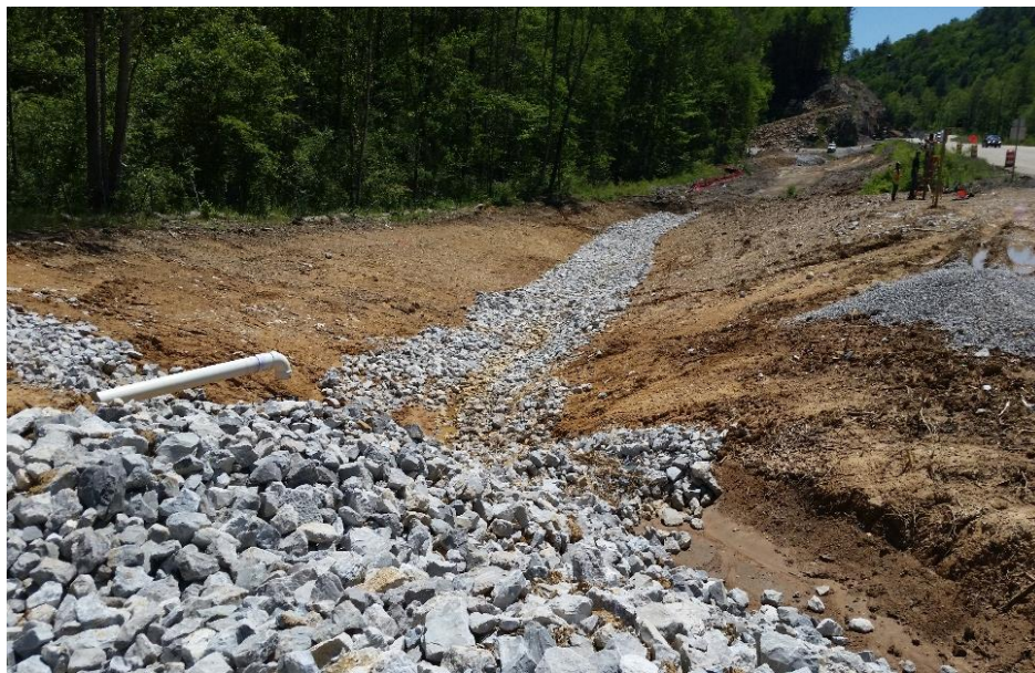
Figure 3-3. Morgan County sediment basin outlet and downstream condition.
