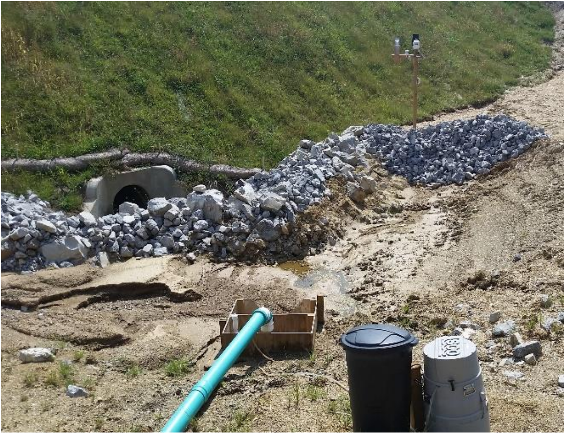
Figure 3-5. Knox County sediment basin outlet pipe and downstream condition.
