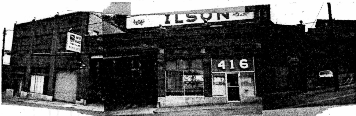
Buildings East of Site - South Side of Jackson Ave.
