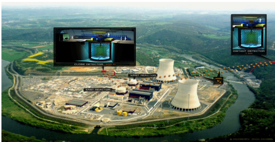
Figure 4.1: Chooz-B nuclear reactor site in northeastern France. Near Lab (~400 from reactor cores) and Far Lab (~1.05km from reactor cores) are shown.
