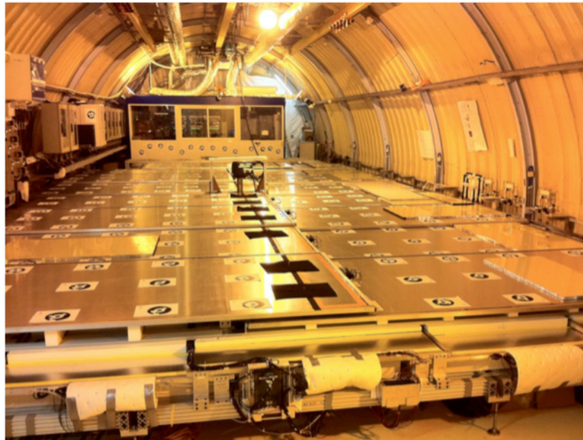
Figure 4.4: Installed lower OV panels.
