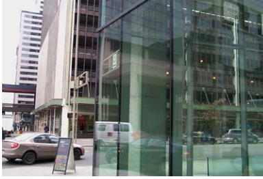
Figure 2.10 Corner cut away of CAC (Author)
