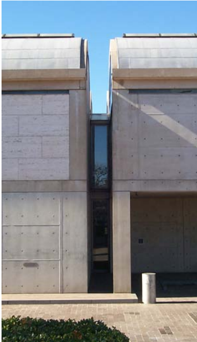
Figure 1.7 Space between Vaults (Author)
