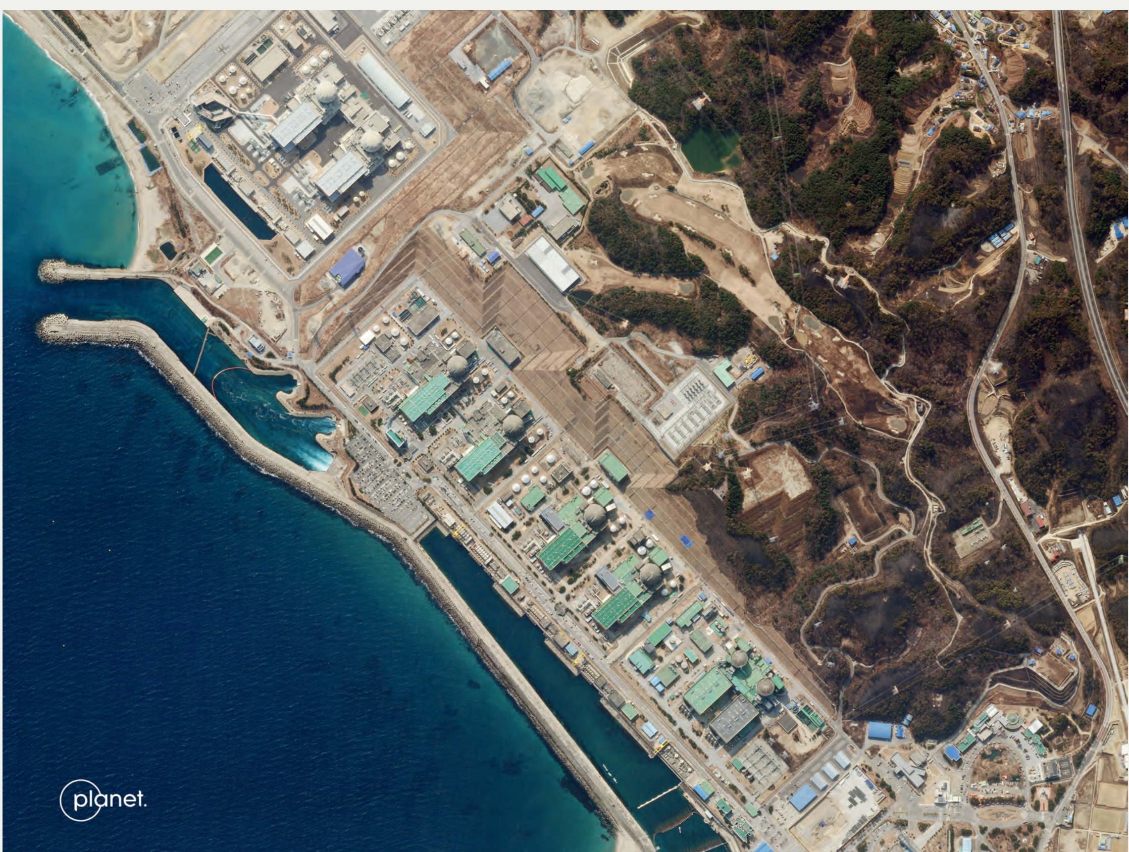
Hanul Nuclear Power Plant (11 March 2022)
