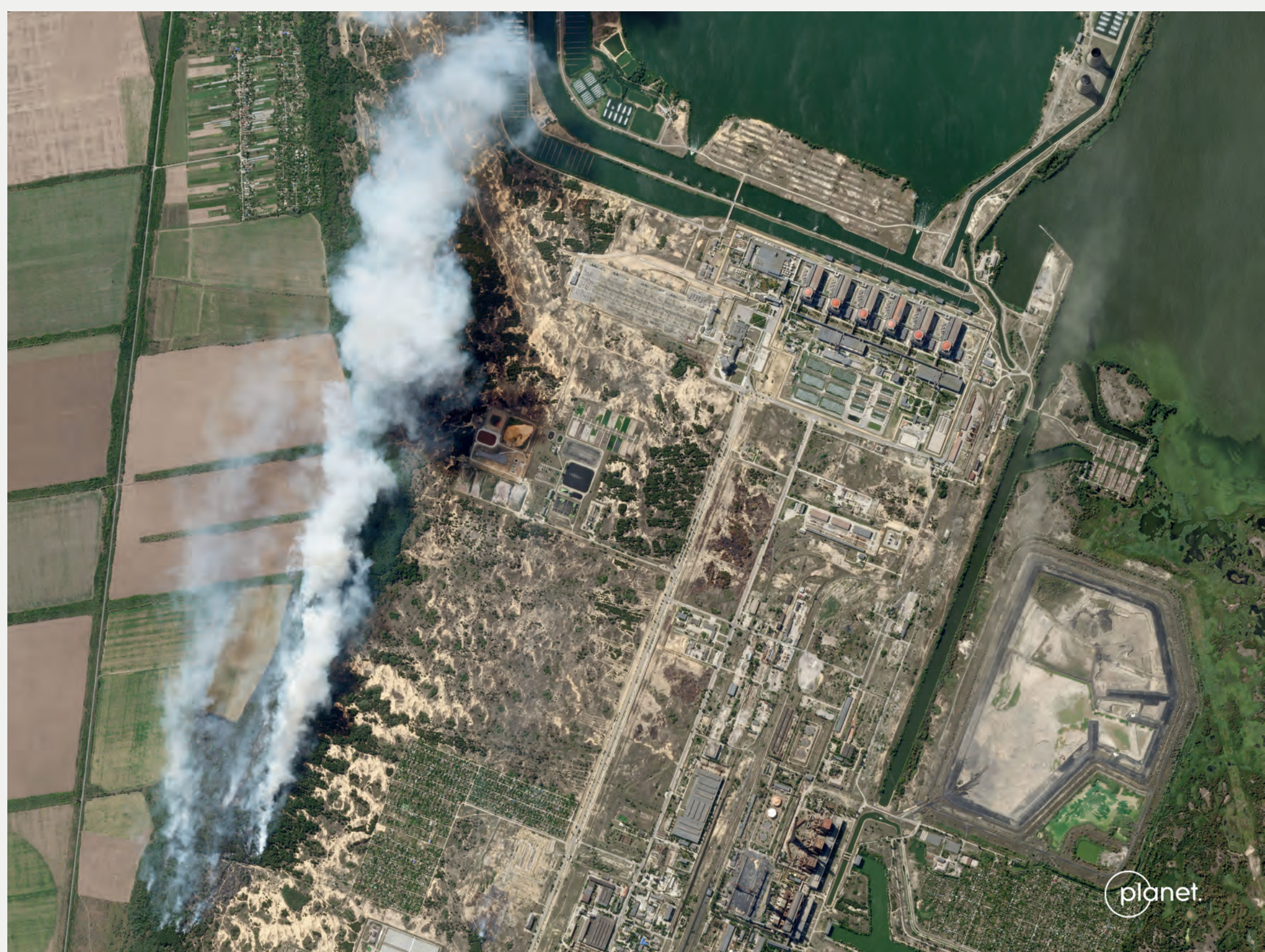
Zaporizhzhia Nuclear Power Plant (26 August 2022)
