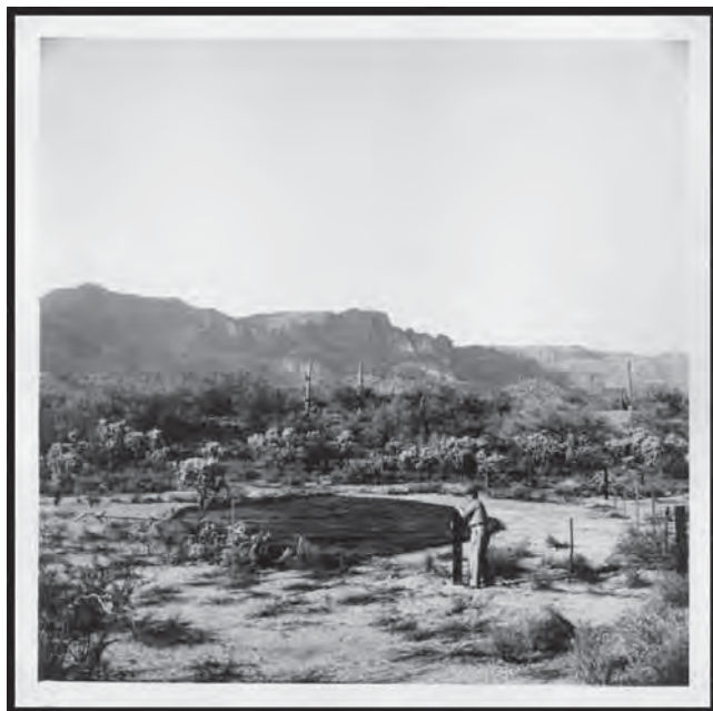
Fig. 3. Tom Kimball showing one of the first quail water catchments in the Superstition Mountains, Arizona, ~1946. The apron of this 'gallinaceous guzzler' is of asphalt and the water capacity of the catchment is limited to a few hundred liters.
