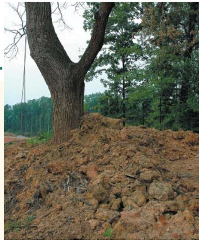
This dozer filling is an example of detrimental grading.
