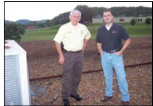
Cannon County Sheriff Darrell Young and Doug Bodary stand atop the county jail prior to the renovation project.
