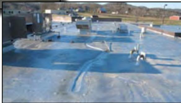
New heating and air conditioning units were installed on the new SPF jail roof.
